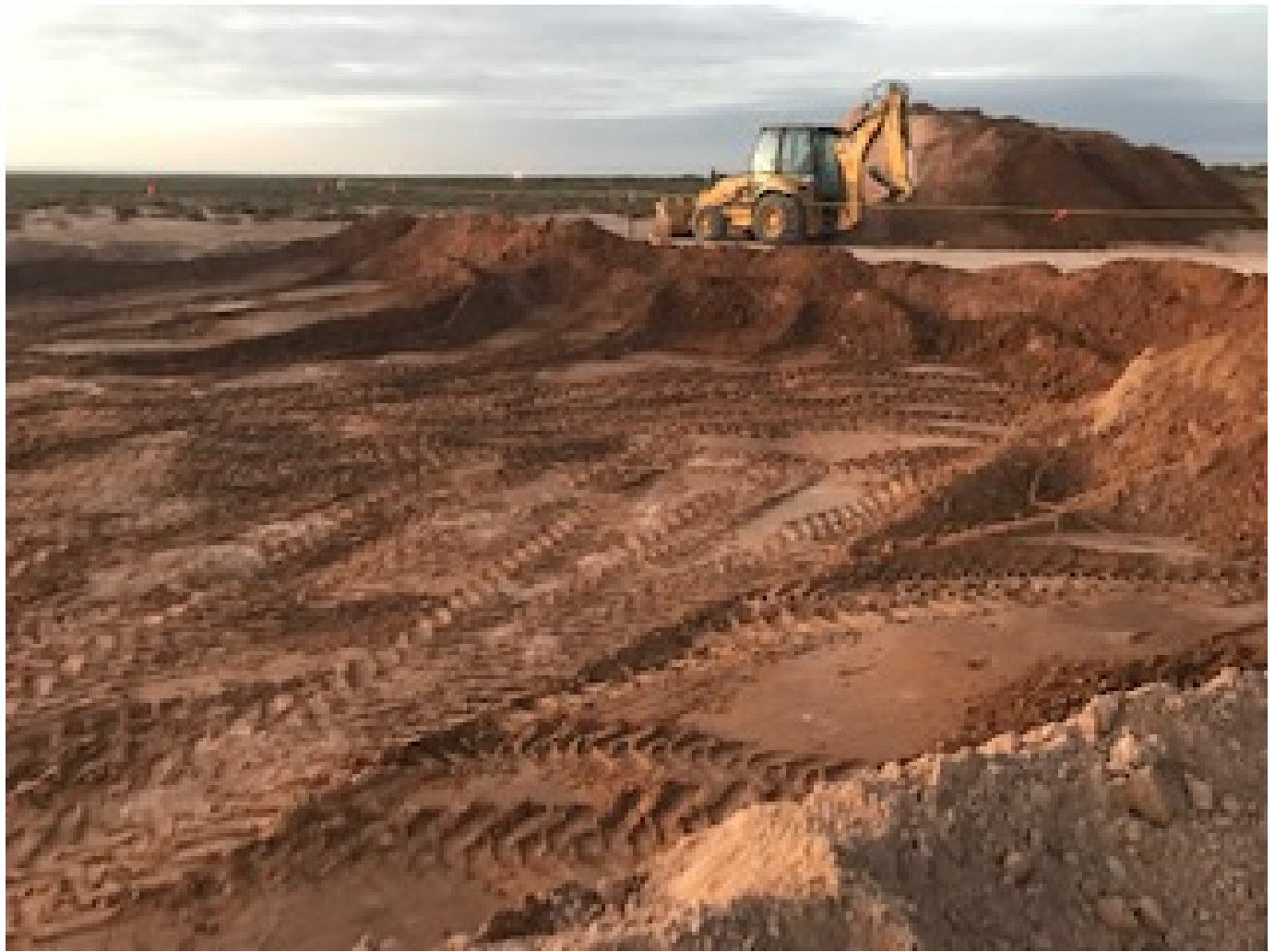
View of the north and western excavation boundaries
