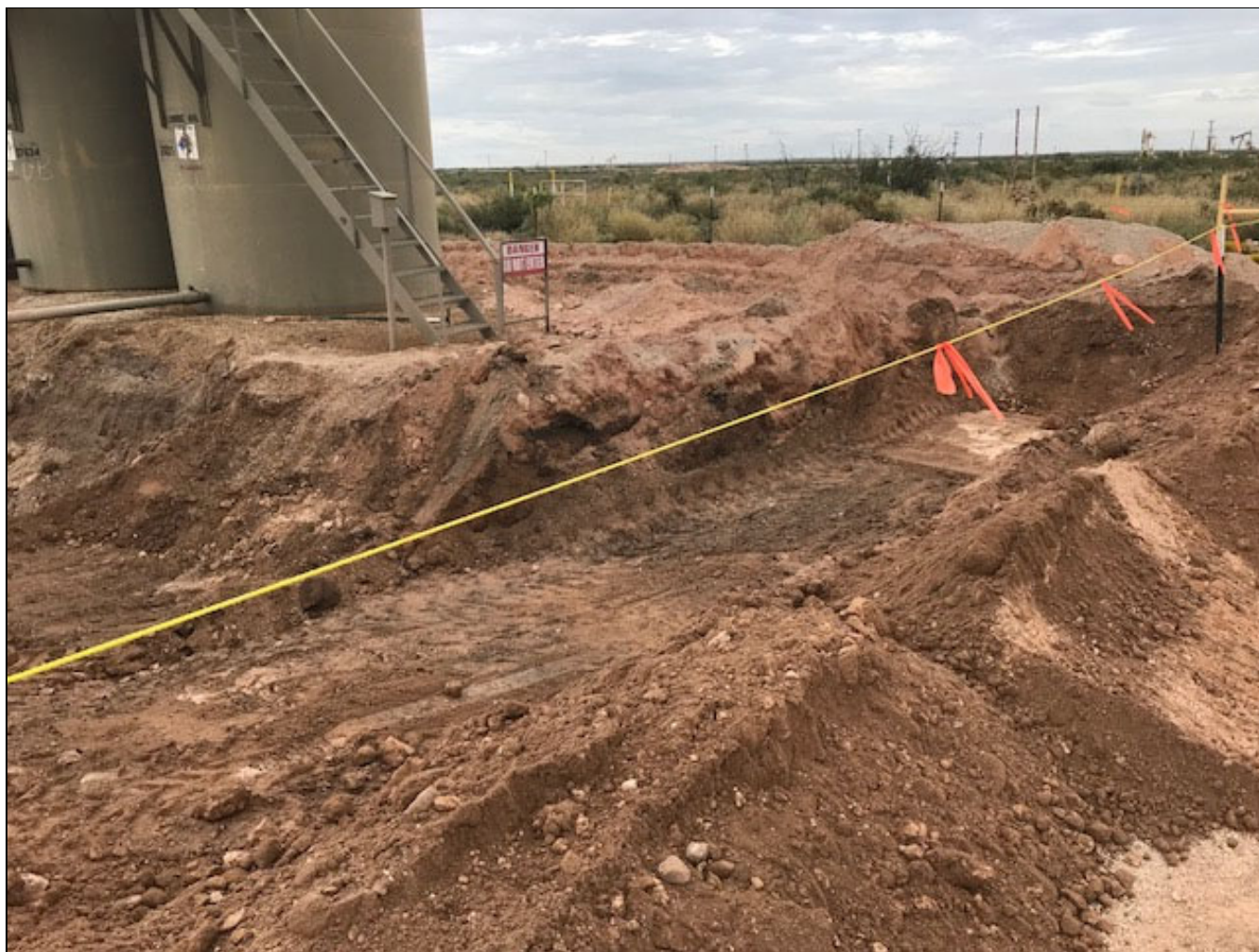
View of the excavation southern boundary
