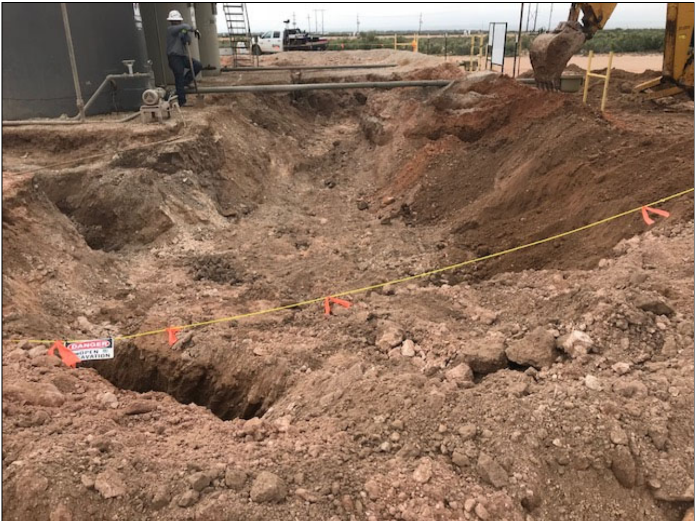
View of the excavation area and tank battery
