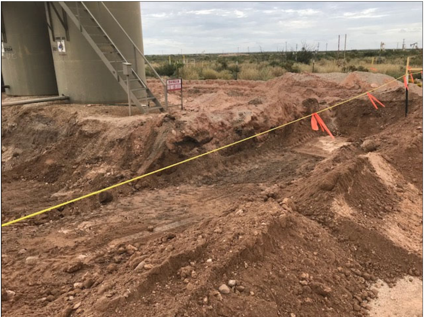
View of the excavation southern boundary
