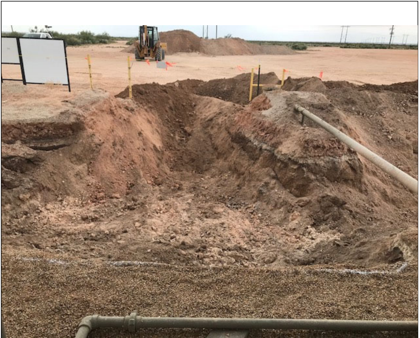
View of product line within excavation
