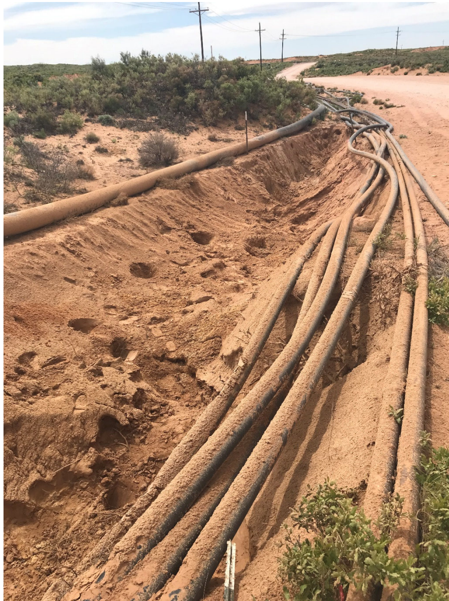
View facing west of the excavation area (2RP-5231).
