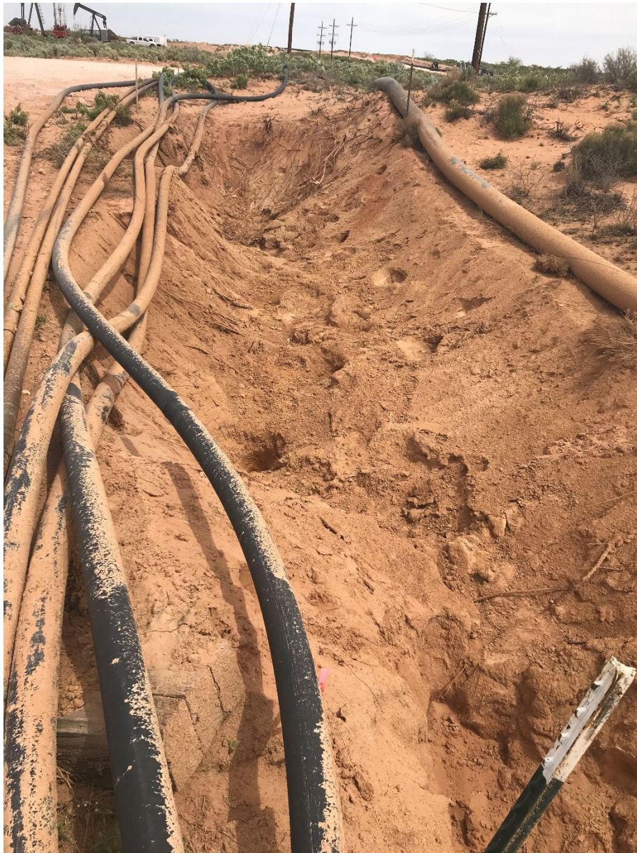
View facing east of the excavation area (2RP-5231).
