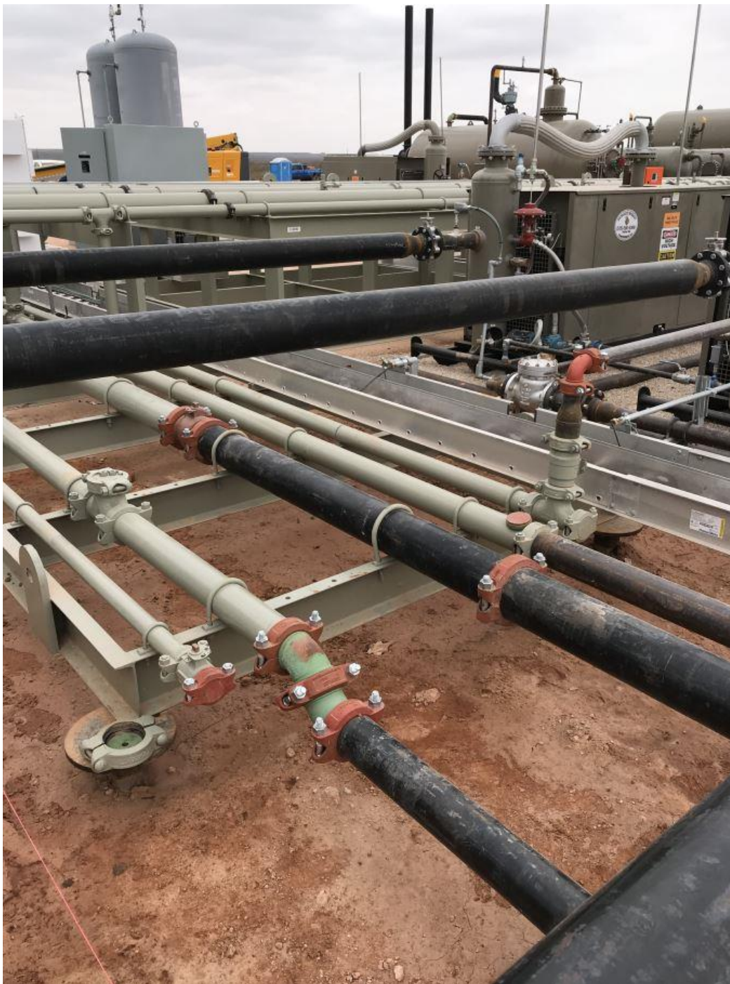
Northeastern view of release area south of processing equipment prior to delineation activities.
