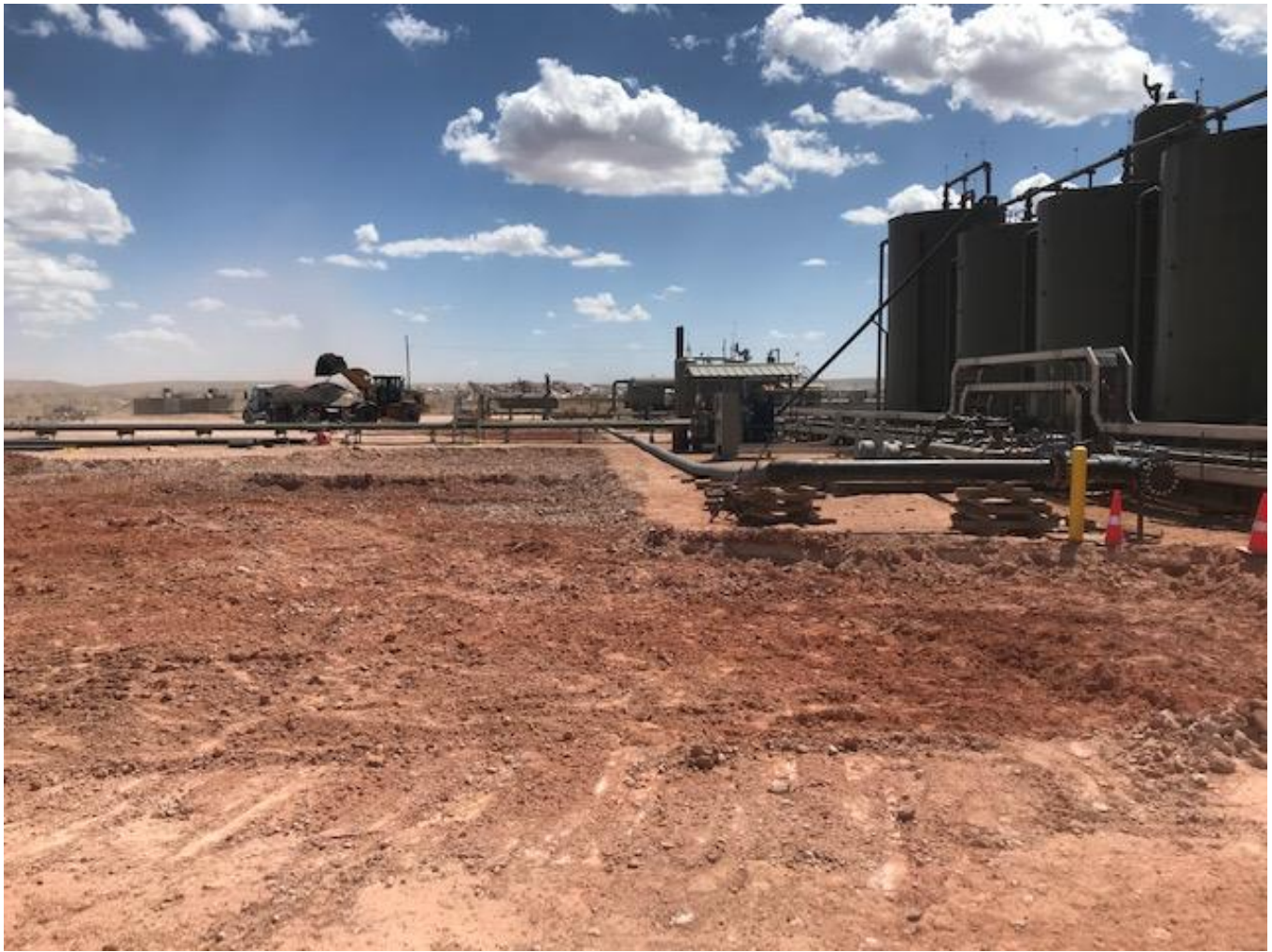
Eastern view of the excavation and active pipelines and processing equipment.
