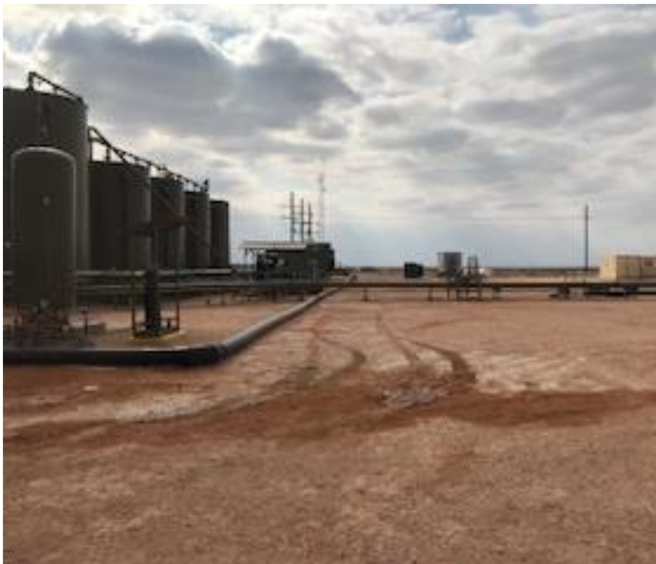
Western view of release area prior to excavation and delineation activities.
