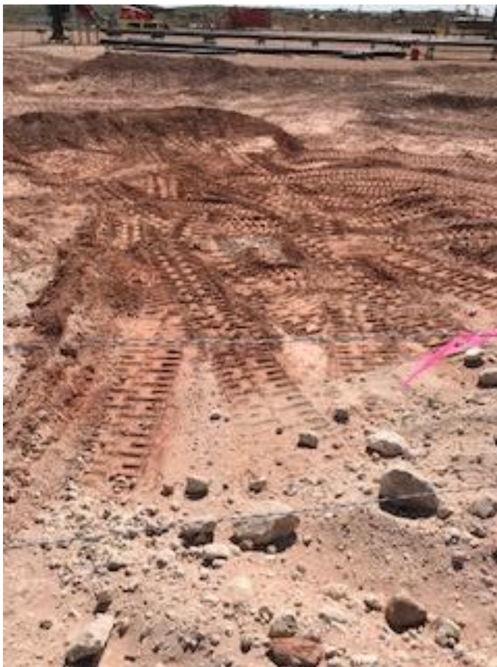
Western view of the final excavation extent on the western edge of the well pad.
