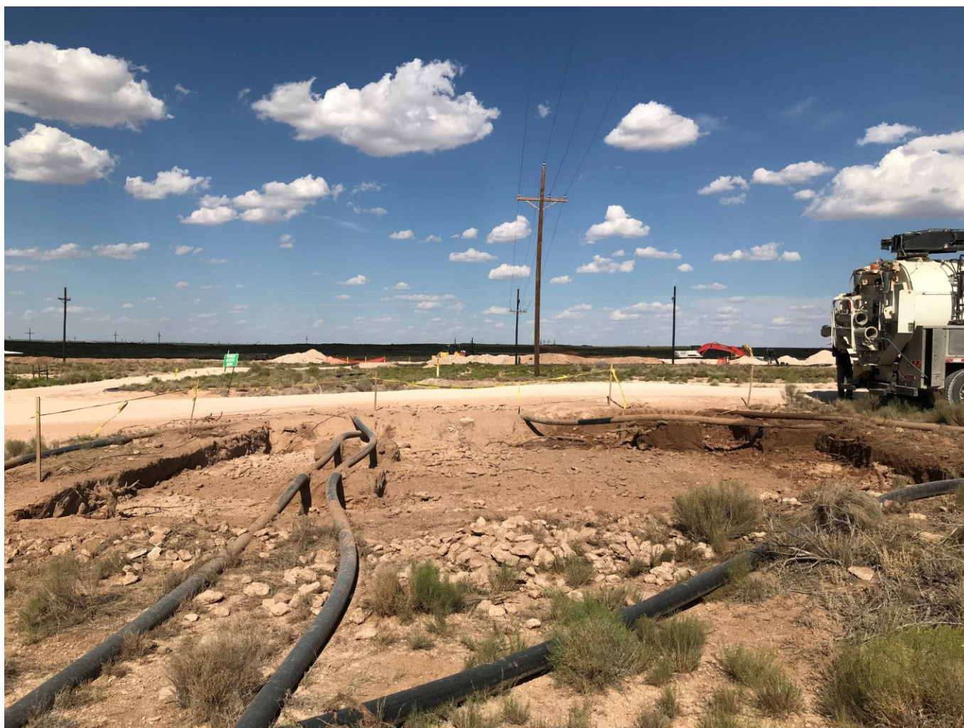
Eastern view of final excavation extent to the west of the lease road.
