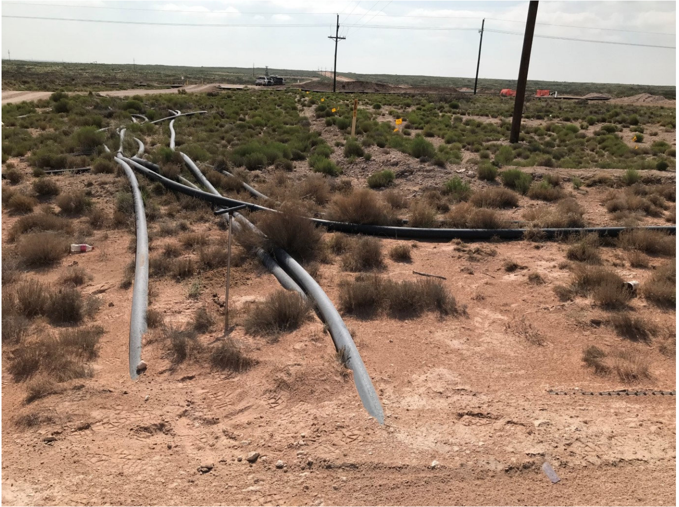
Eastern view of point of release identified on flow line during site assessment.
