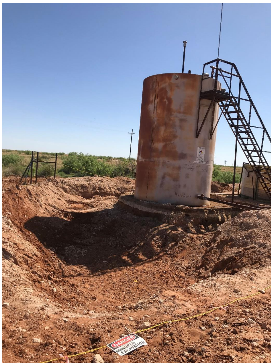
View facing south during excavation activities.
