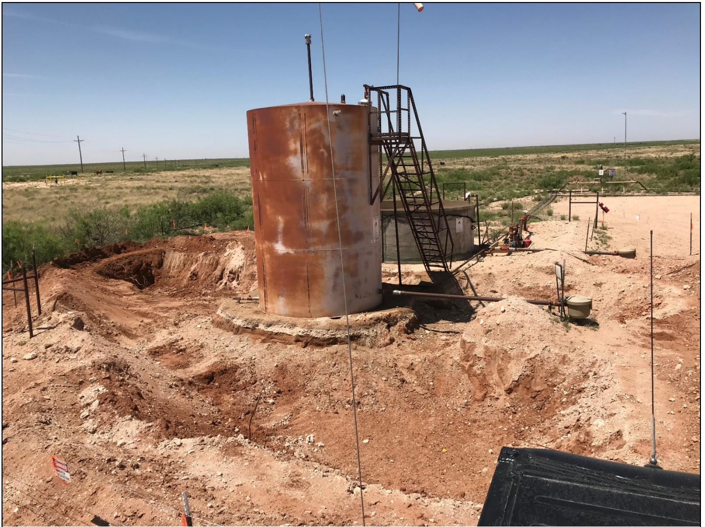
View facing southwest during excavation activities.
