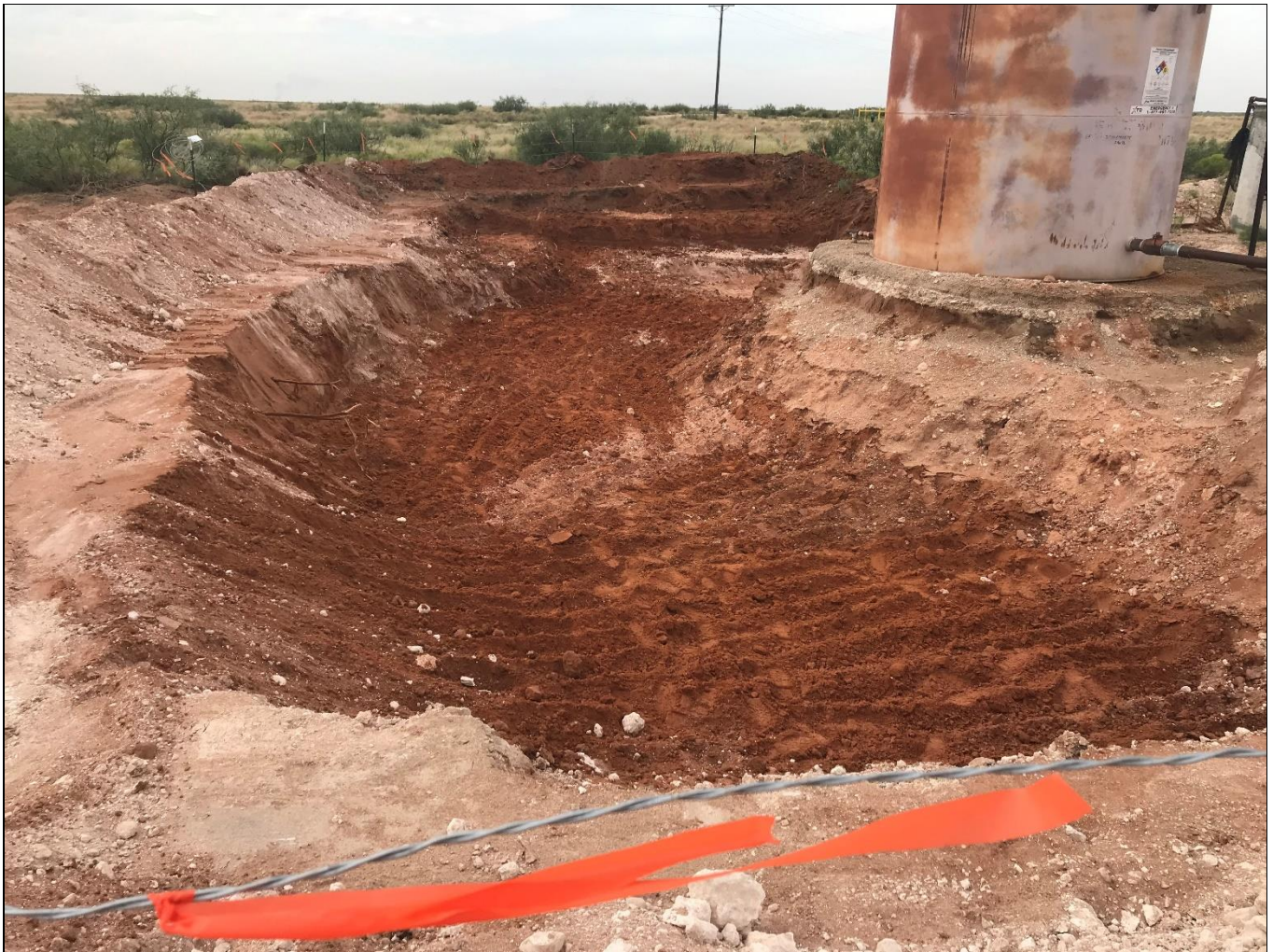
View facing north of the final excavation extent.
