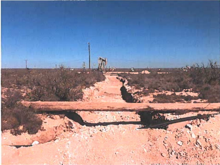
Photo of Two Foot Excavation Facing North 11/19/18
