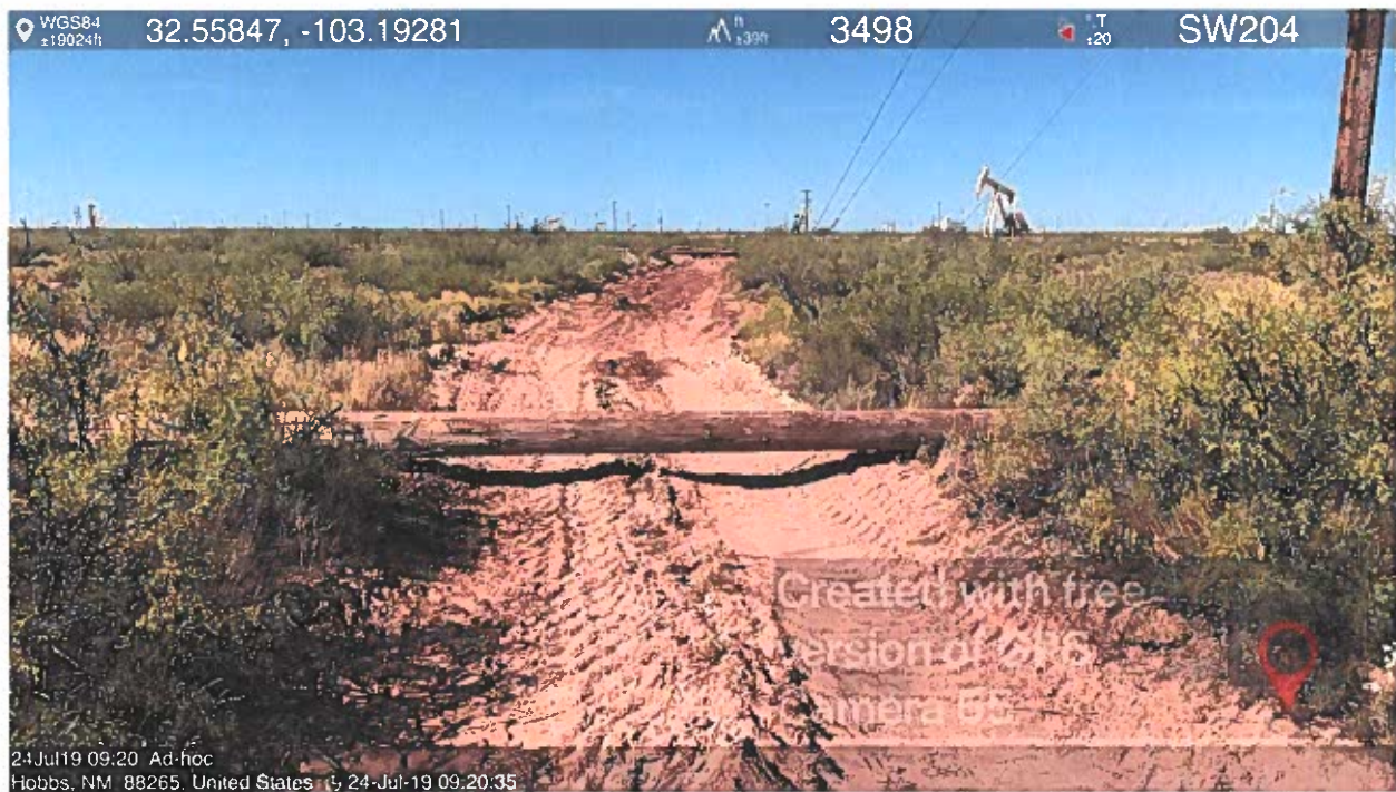
Photo of Pasture Area Backfilled 7/24/19
