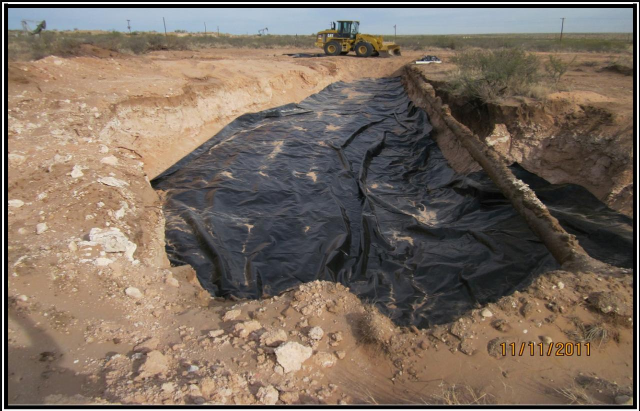
View of the west terminus of the release after installation of liner.
