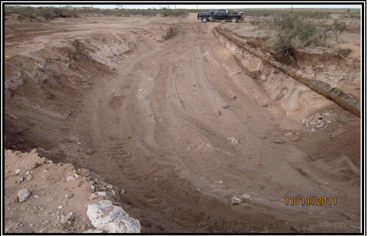
View of the west terminus of the release after backfill emplaced over liner.
