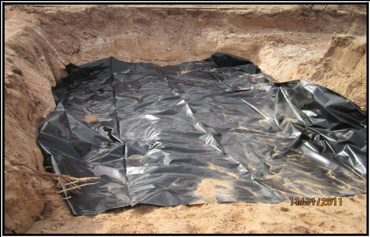
View of east terminus of the release after installation of liner.
