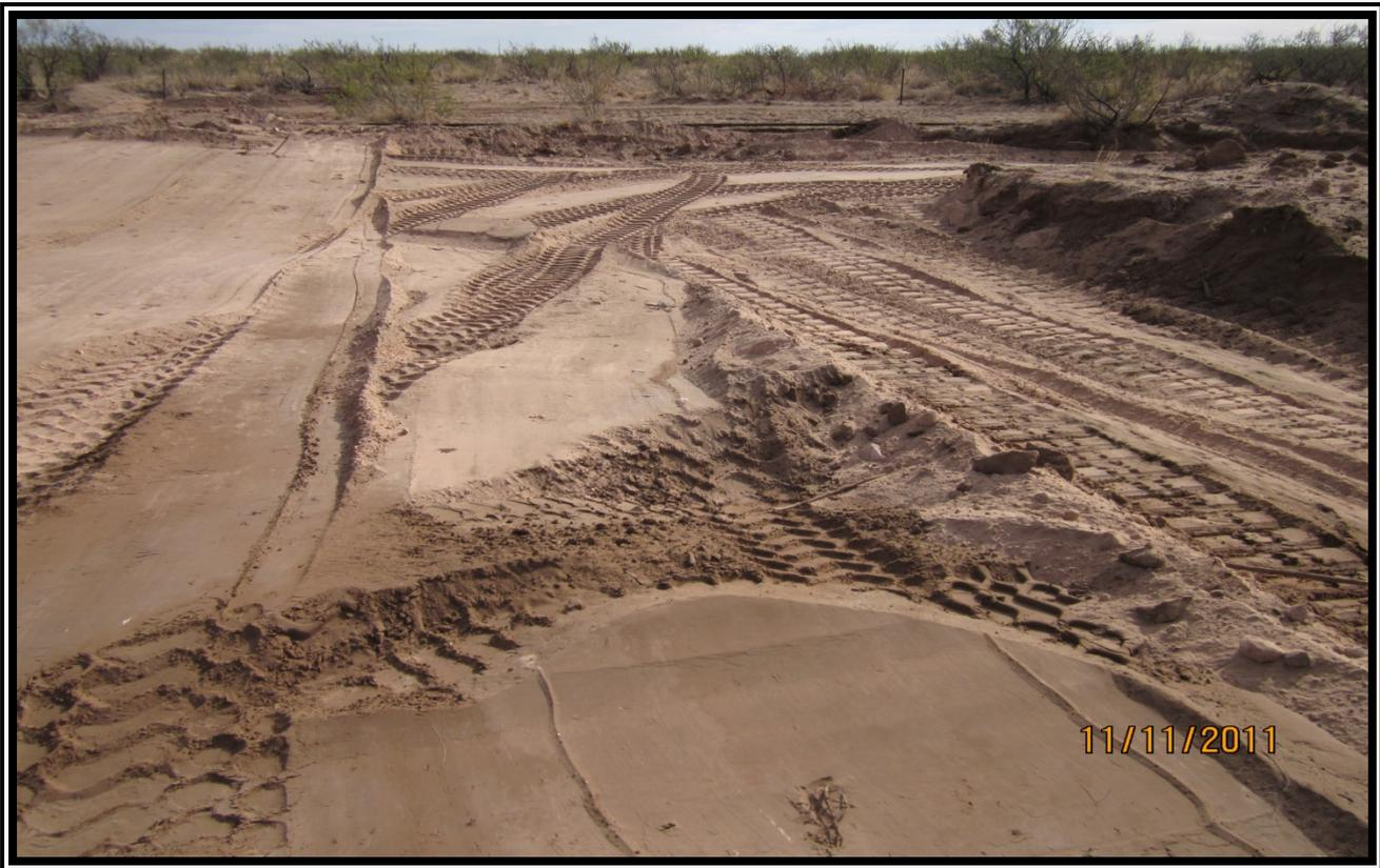
View of east terminus of the release after backfill emplaced over liner.
