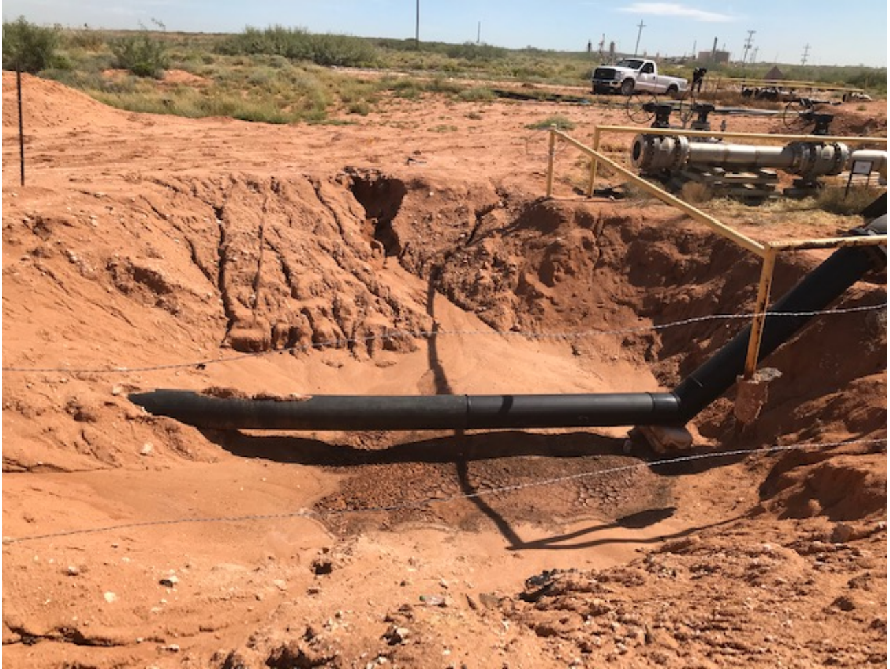
Existing excavation from recently exposing the riser and release facing north during Site assessment activities.
