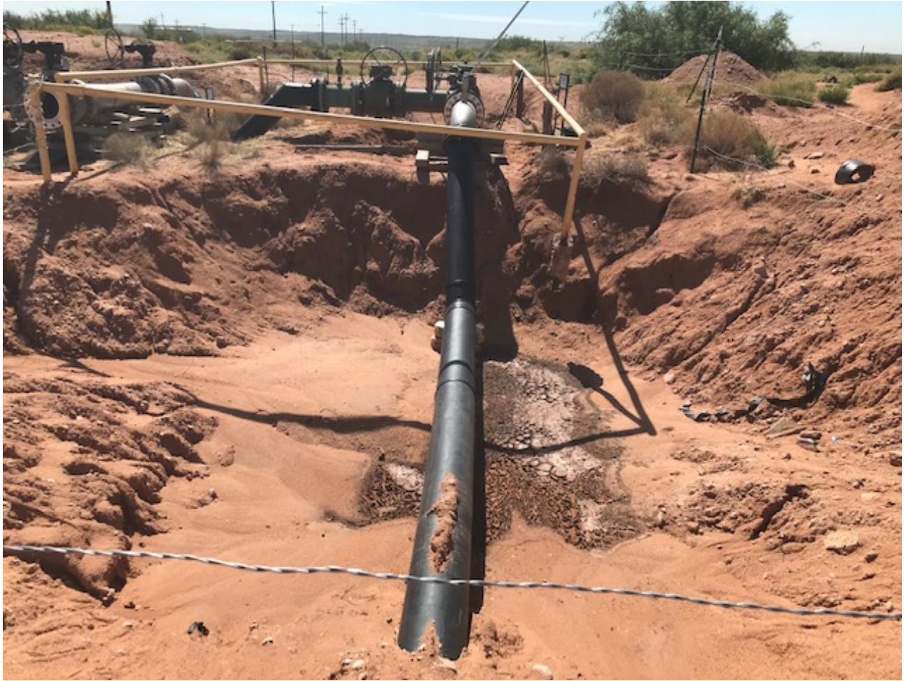
Existing excavation from recently exposing the riser and release facing east during Site assessment activities.
