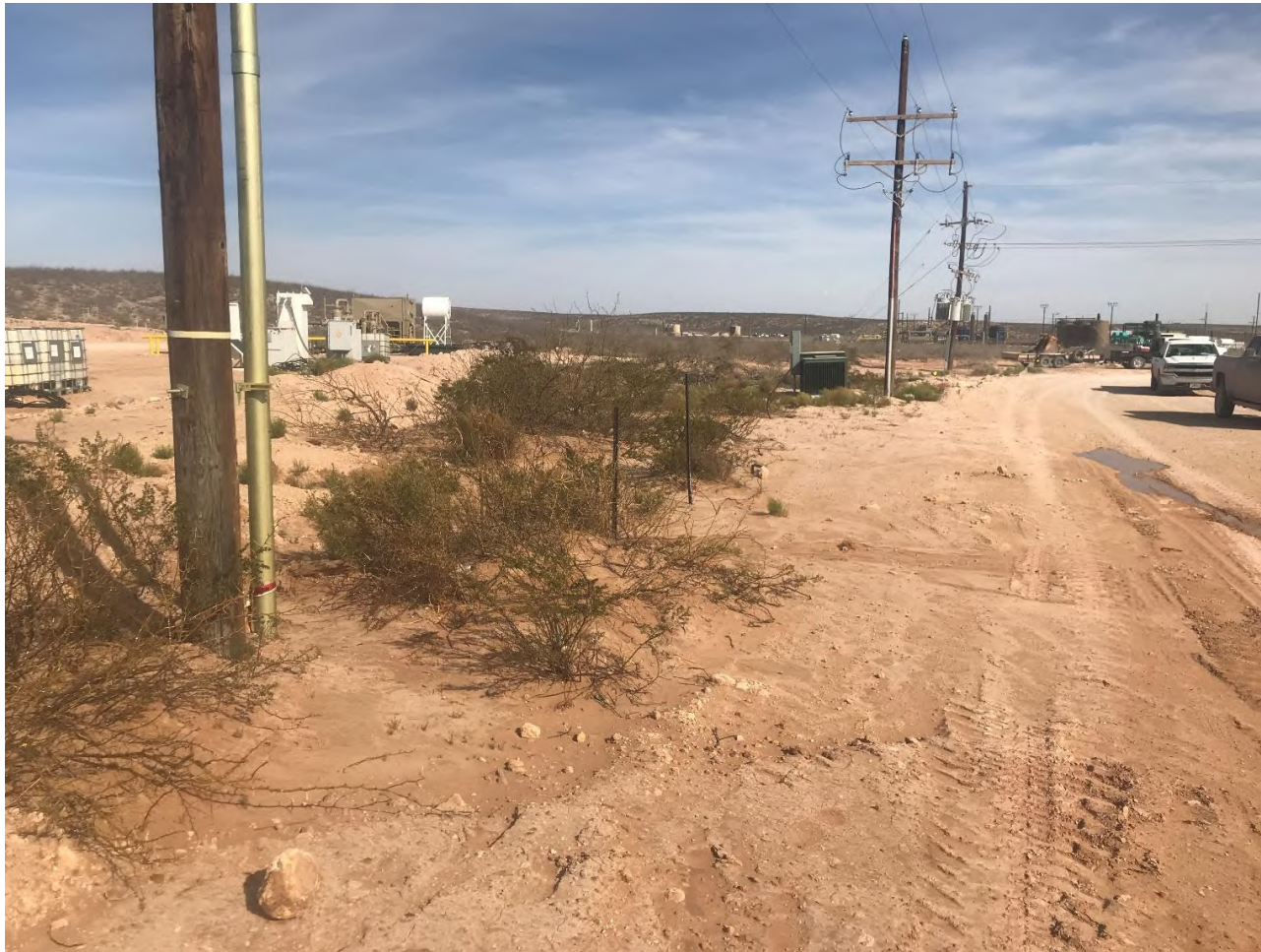
Northern view of release area and ROW during site assessment activities.
