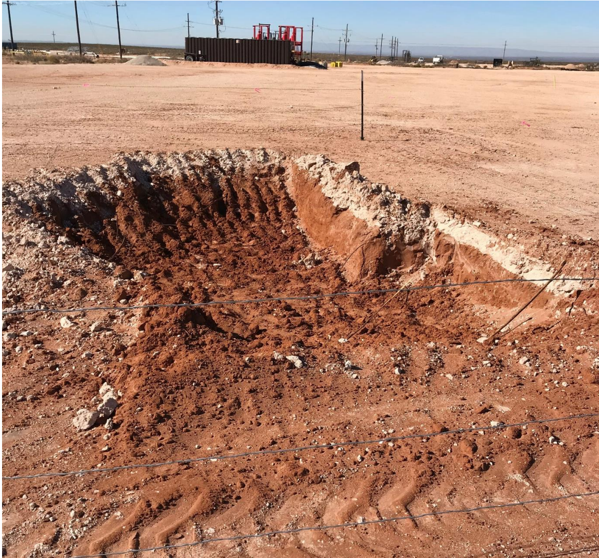
Northwestern view of final excavation extent during confirmation soil sampling activities.
