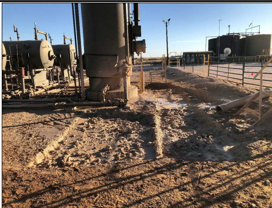
PHOTO 12: View of hydrovac excavating activity near release source facing south. 11/18/19
