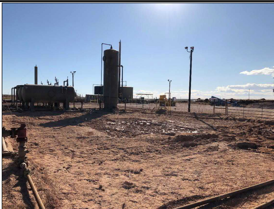
PHOTO 22: View of hydrovac excavating activity inside containment facing south-southwest. 11/21/19
