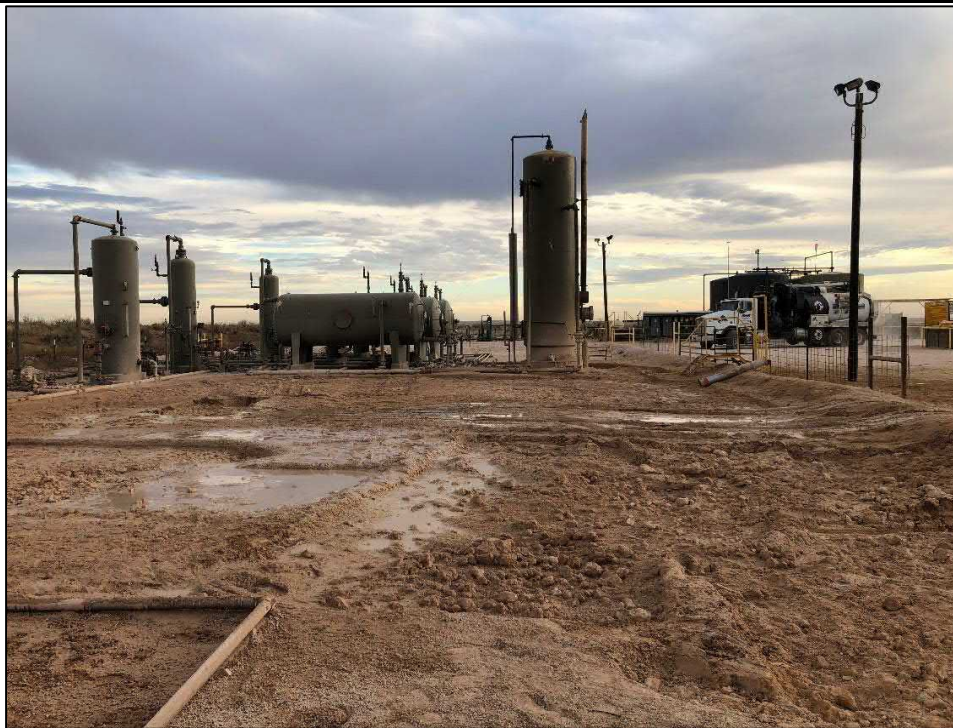
PHOTO 13: View of hydrovac excavating activity facing south. 11/19/19
