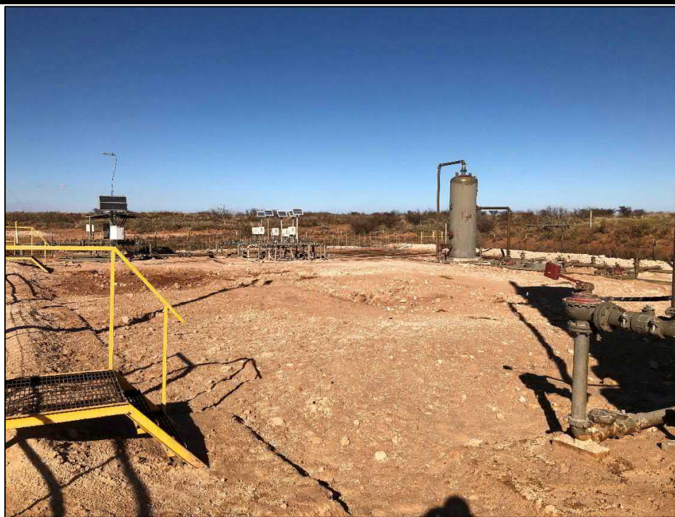
PHOTO 21: View of hydrovac excavating activity inside containment facing northeast. 11/21/19
