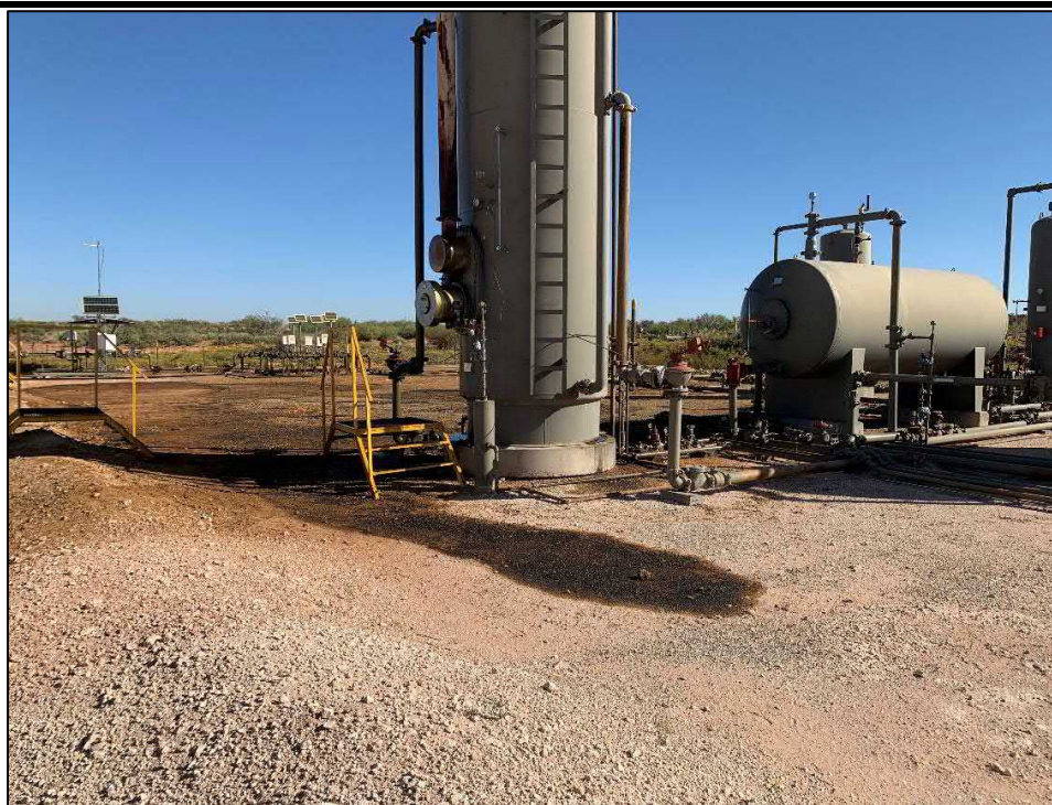
PHOTO 2: View of fluid release area inside containment facing north-north east. 10/17/19
