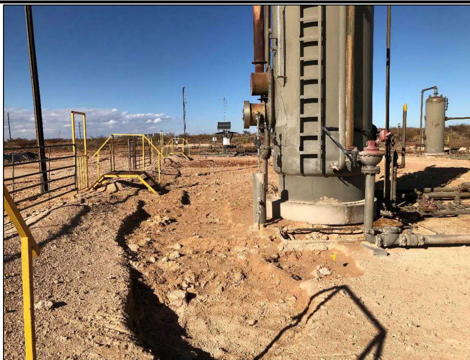
PHOTO 20: View of hydrovac excavating activity inside containment facing north. 11/21/19
