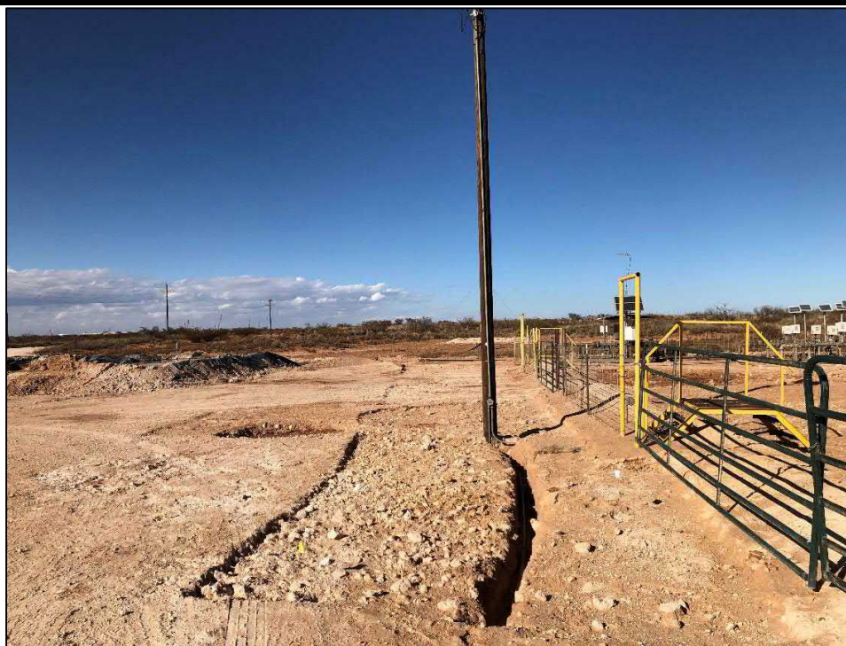
PHOTO 19: View of hydrovac excavating activity outside containment facing north. 11/21/19
