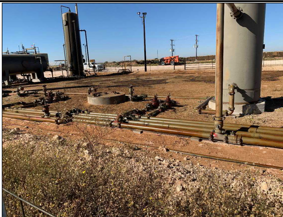
PHOTO 8: View of over spray area inside containment facing southwest. 10/17/19
