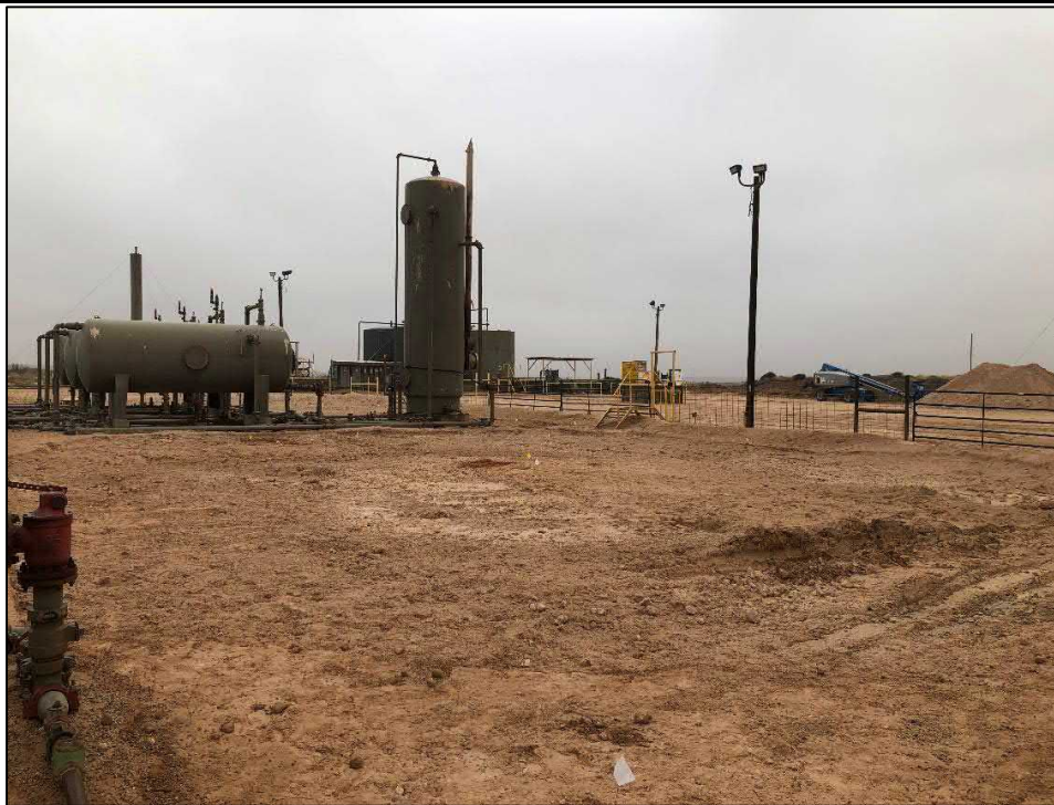
PHOTO 17: View of hydrovac excavating activity facing southwest. 11/20/19
