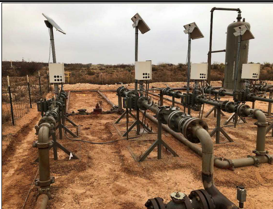
PHOTO 16: View of hydrovac excavating activity around piping facing east. 11/20/19
