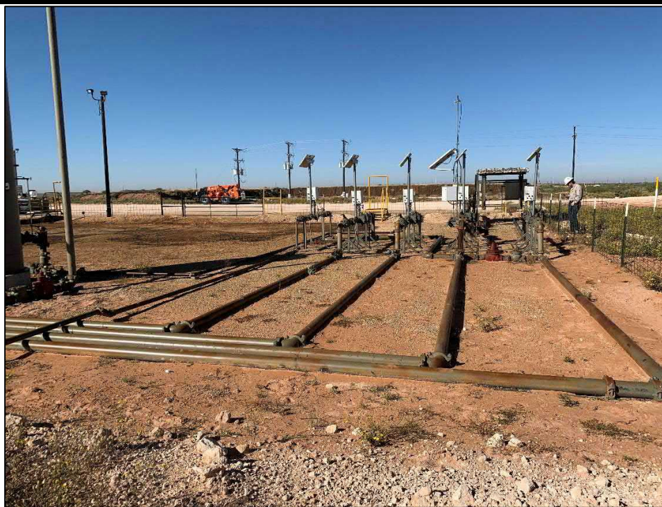
PHOTO 7: View of over spray area inside containment facing west. 10/17/19
