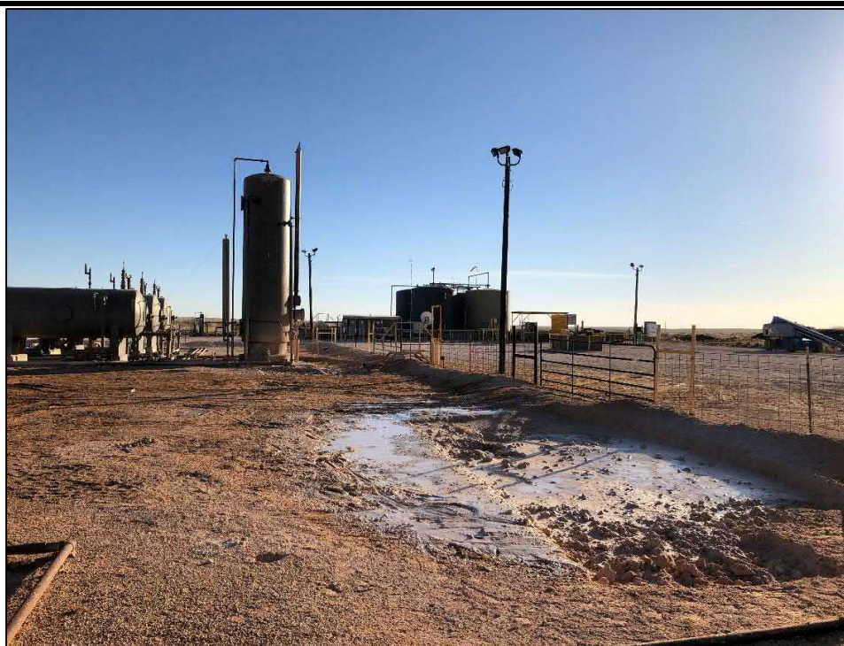
PHOTO 10: View of hydrovac excavating activity facing south. 11/18/19
