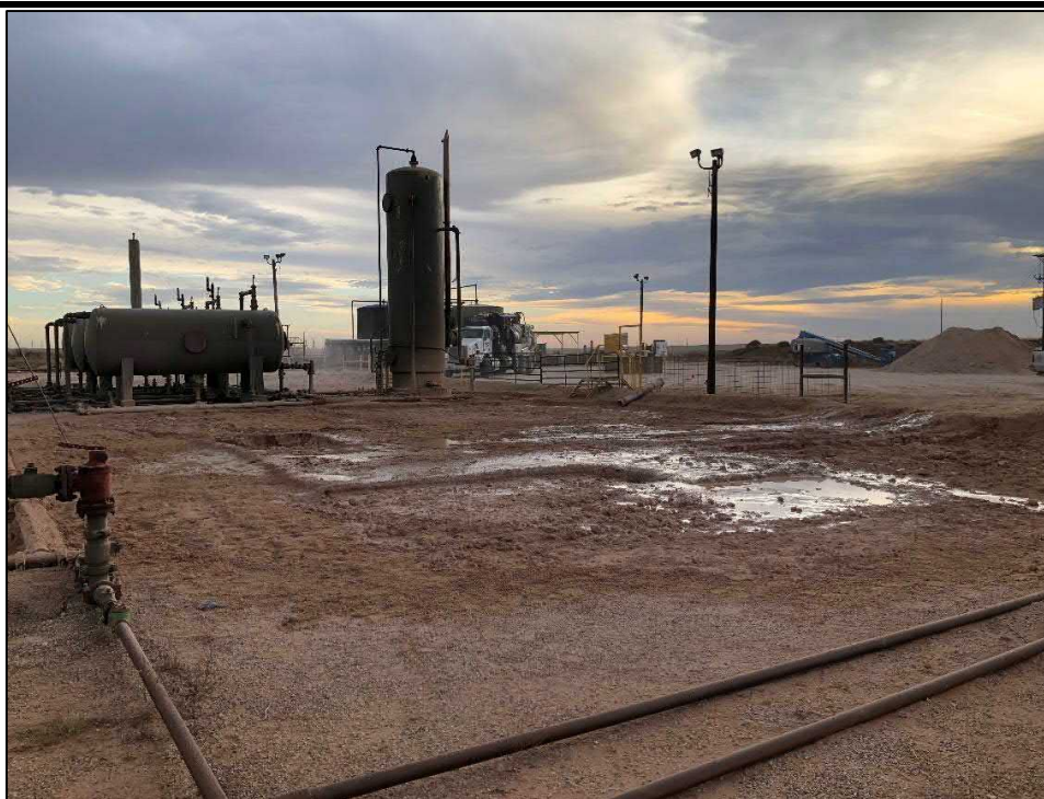
PHOTO 14: View of hydrovac excavating activity facing south-south west. 11/19/19
