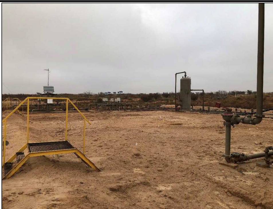
PHOTO 18: View of hydrovac excavating activity facing north-northeast. 11/20/19
