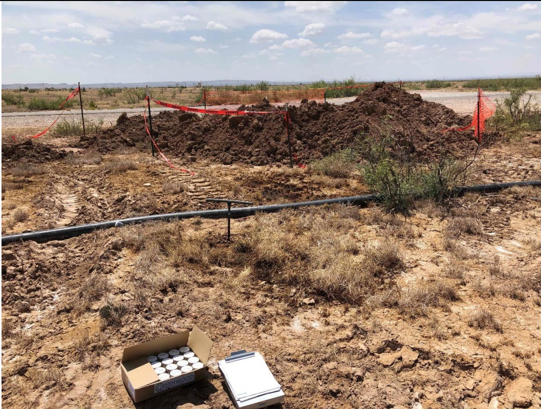
PHOTO 5: View of HA-6, facing south. 8/14/2019
