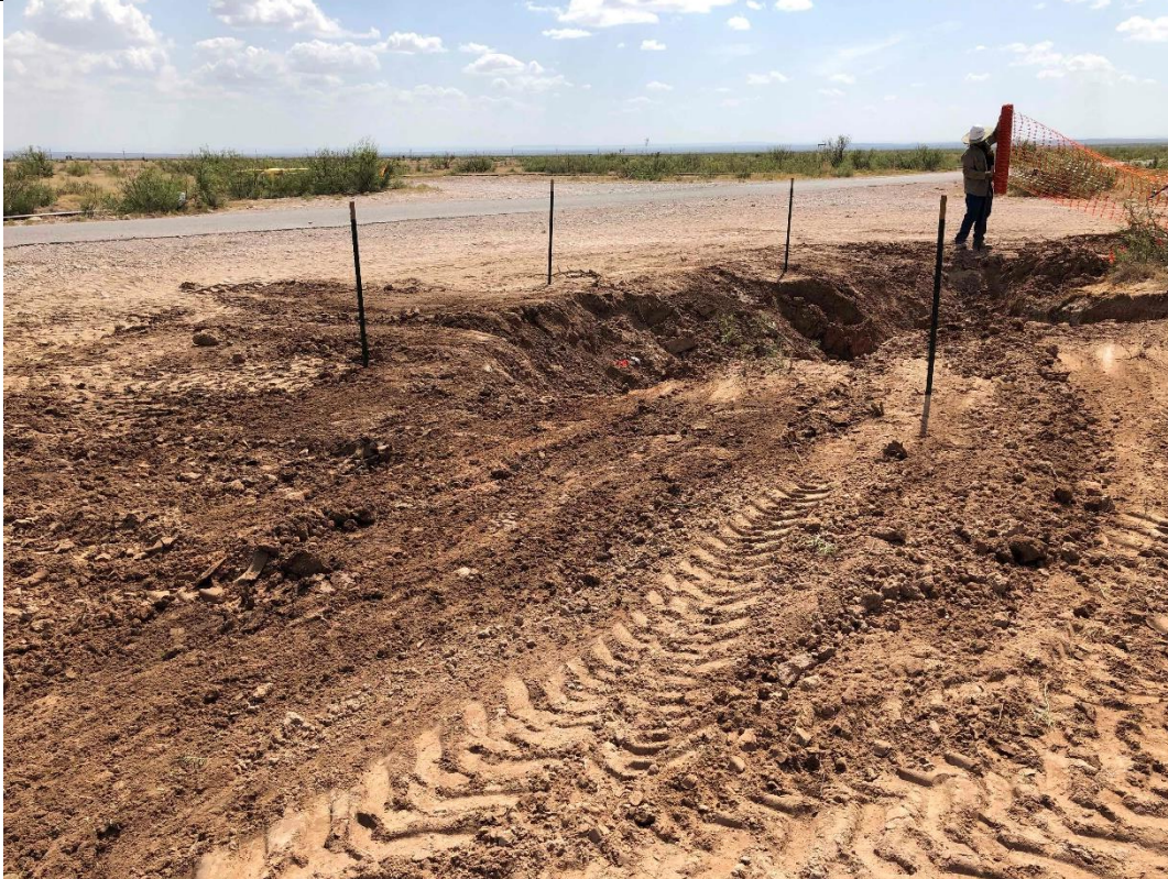
PHOTO 2: View of site securing, facing west. 8/14/2019
