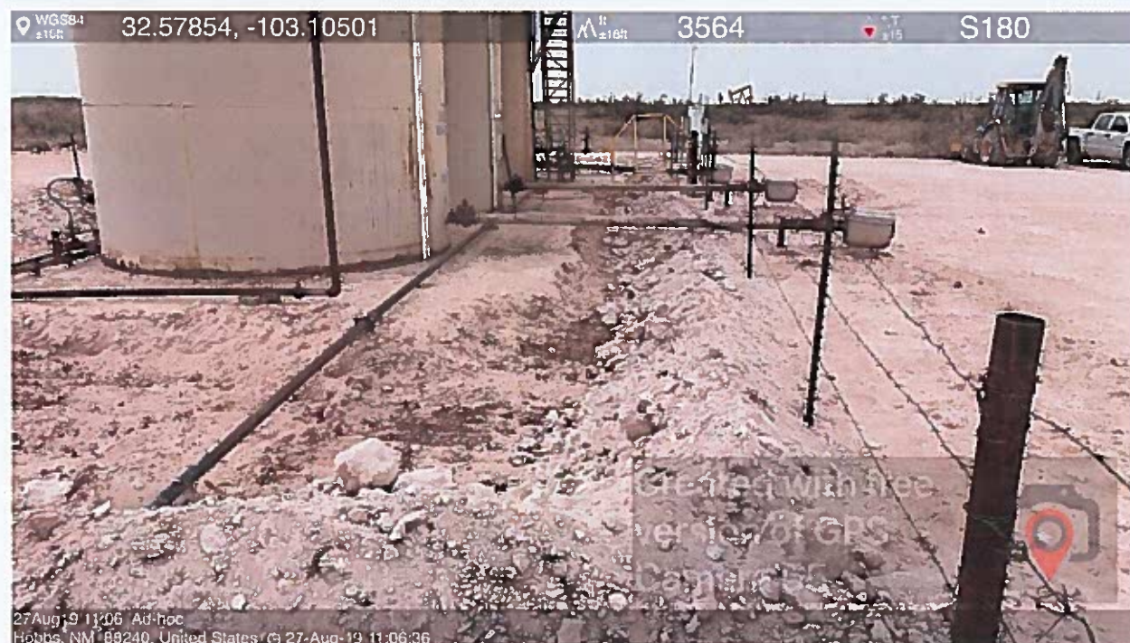
Area excavated with new installed berm
