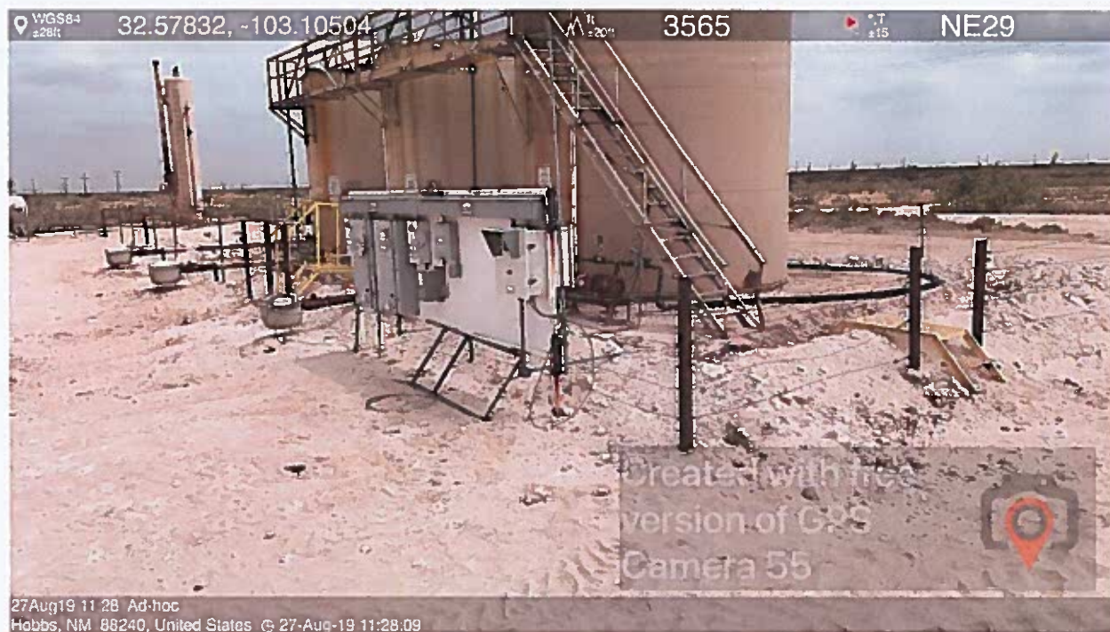
Area excavated with new installed berm
