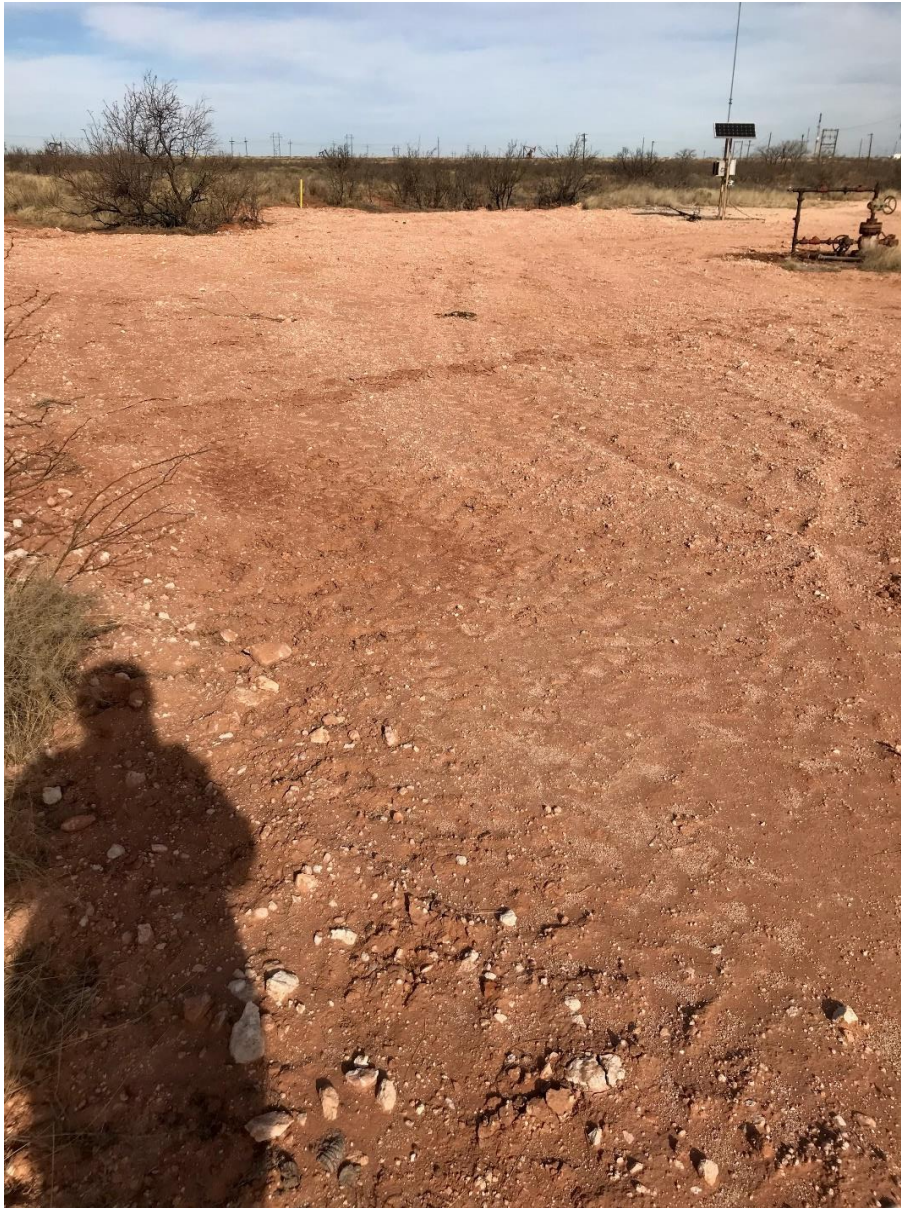
Northern view of backfilled excavation and liner area after delineation and excavation activities.
