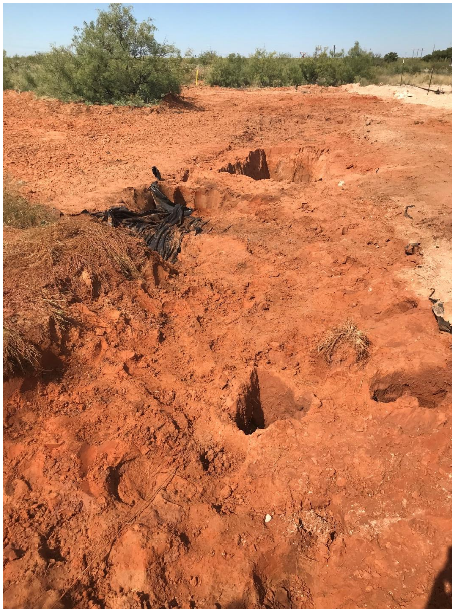
Northern view of liner area during excavation activities.
