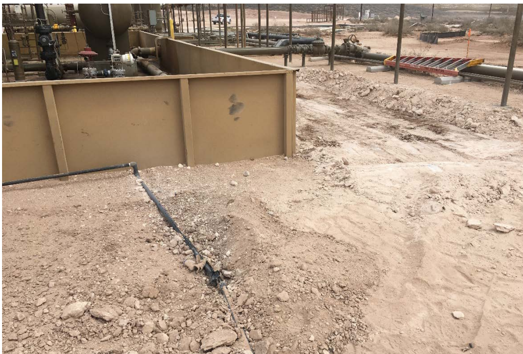
Photograph 2: View of excavation area.
