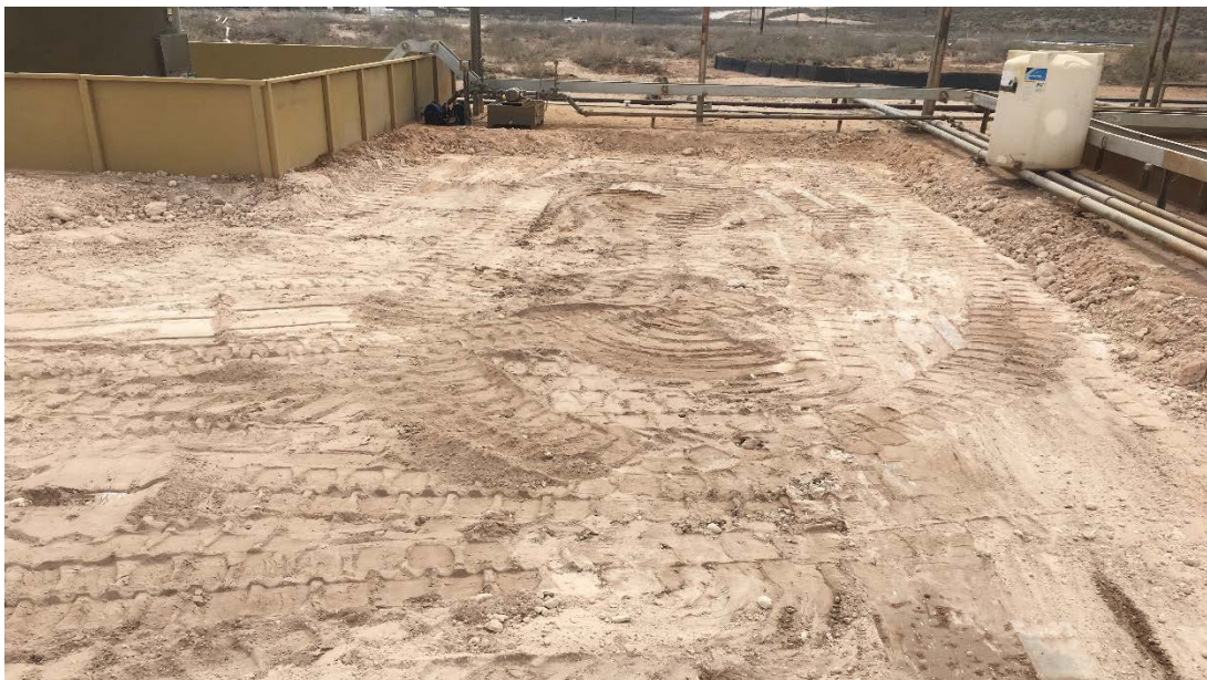
Photograph 3: View of excavation area.
