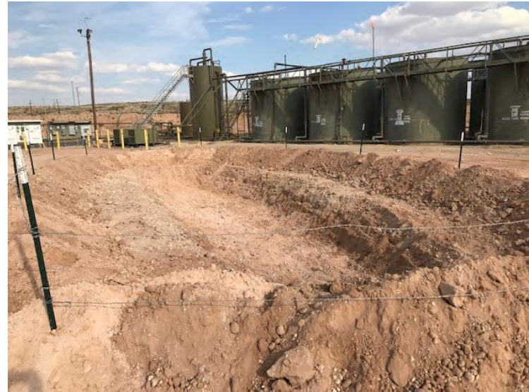
Photograph 2: East facing view of open excavation north of the tanks.
