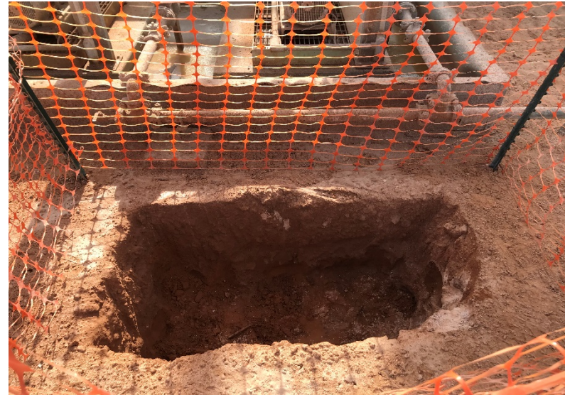
Photograph 2: View of northwest excavation.
