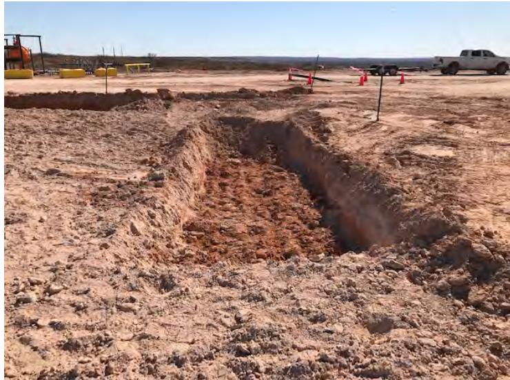
Photograph 3: Southern view of excavation extent.
