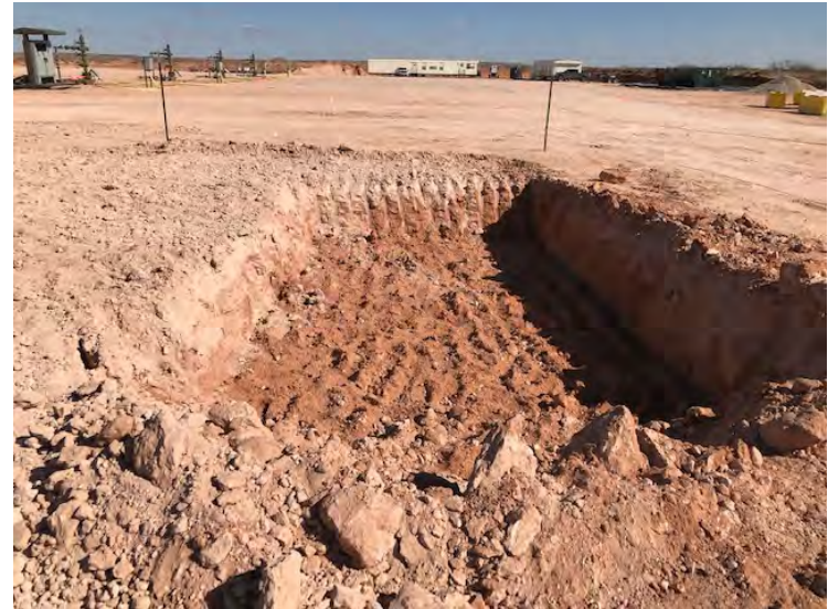
Photograph 4: Western view of excavation extent.
