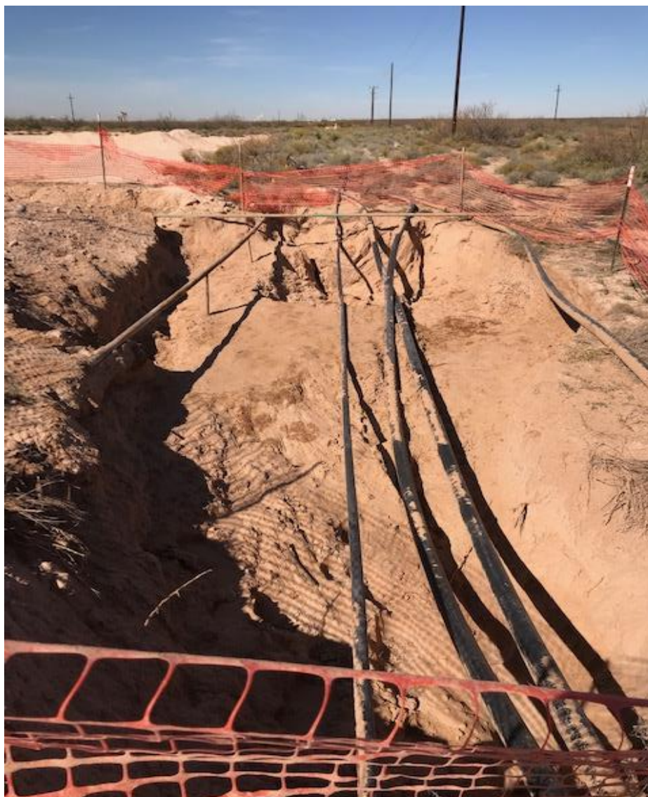
Excavation area – view north
