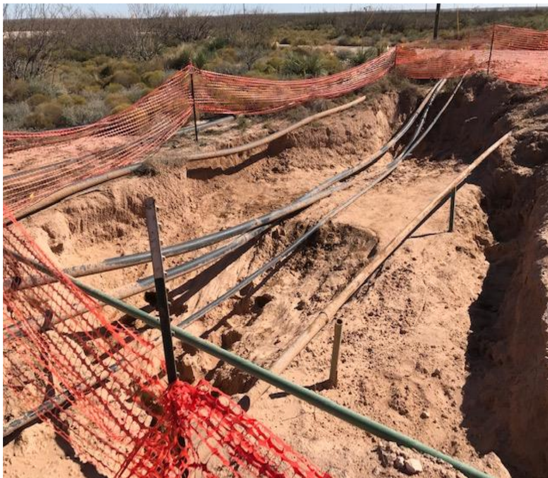
Excavation area – view southeast
