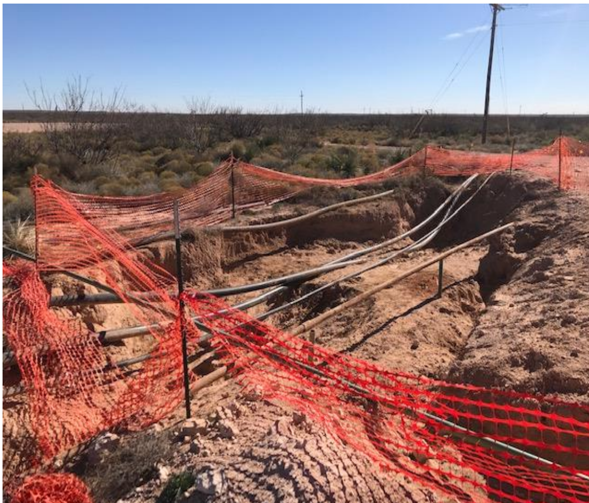
Excavation area – view southeast
