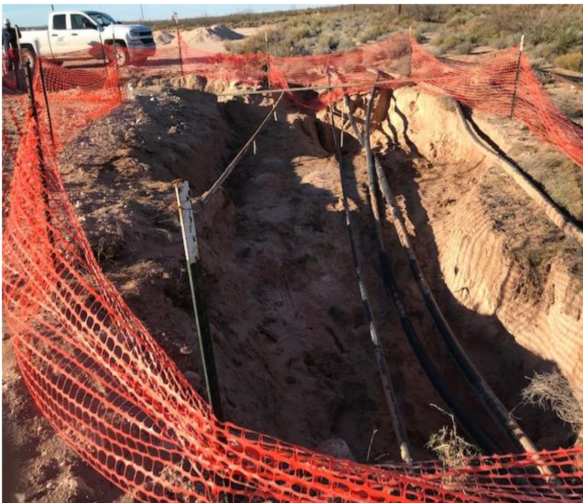
Excavation area – view north
