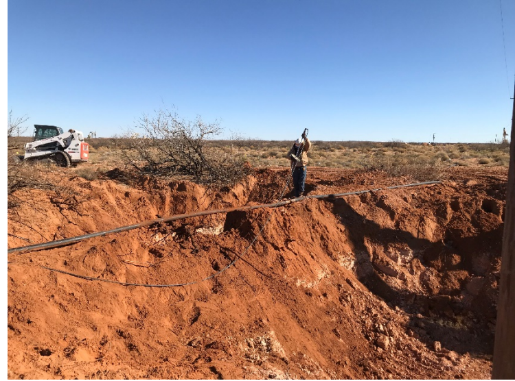
Photograph 2: View north of excavation during hydro-excavation.
