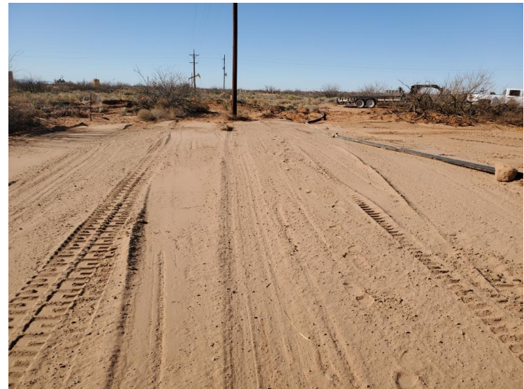
Photograph 4: View west of backfill prior to reseeding.
