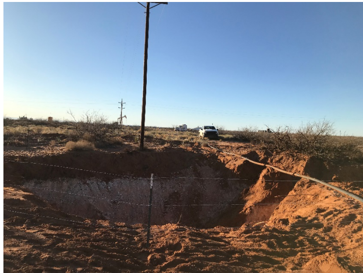
Photograph 3: View west of final excavation extent.
