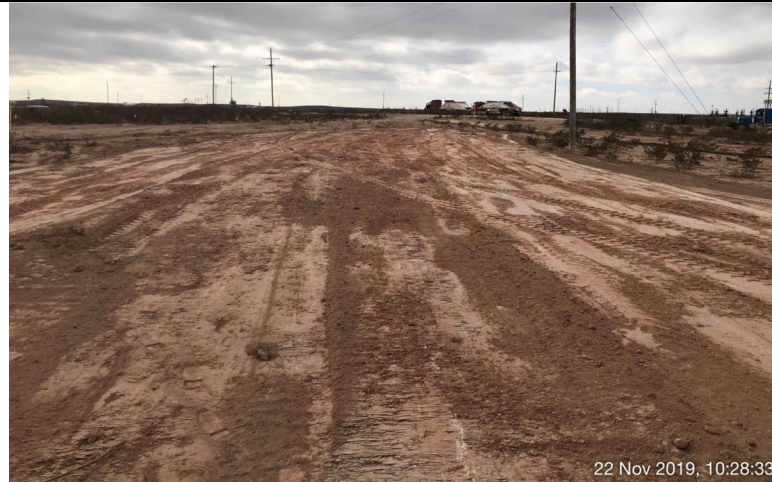
Photo 5: Backfilled area A.
