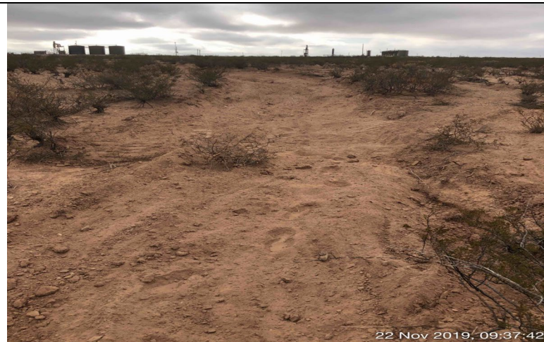
Photo 11: Backfilled area D.
