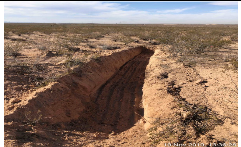
Photo 8: Excavated area C.
