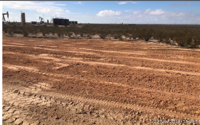
Photo 7: Backfilled area B.
