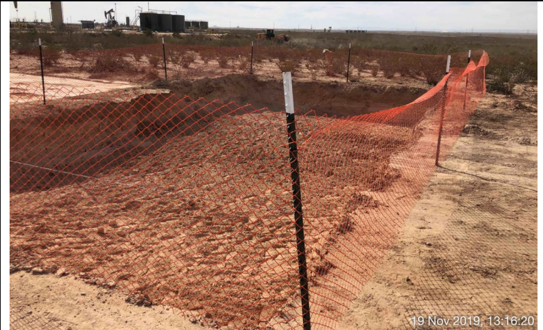
Photo 6: Excavated area B.
