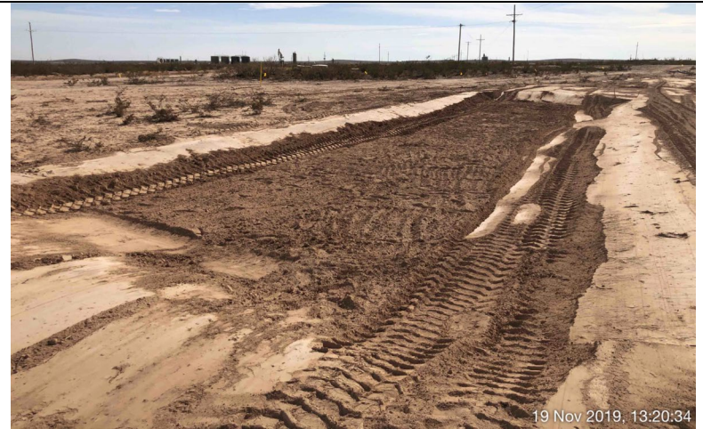
Photo 4: Excavated area A.
