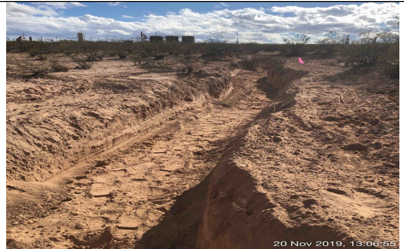
Photo 10: Excavated area D.
