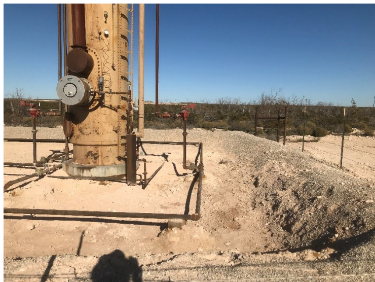
Photograph 5: Southeastern end of the unlined secondary containment.
