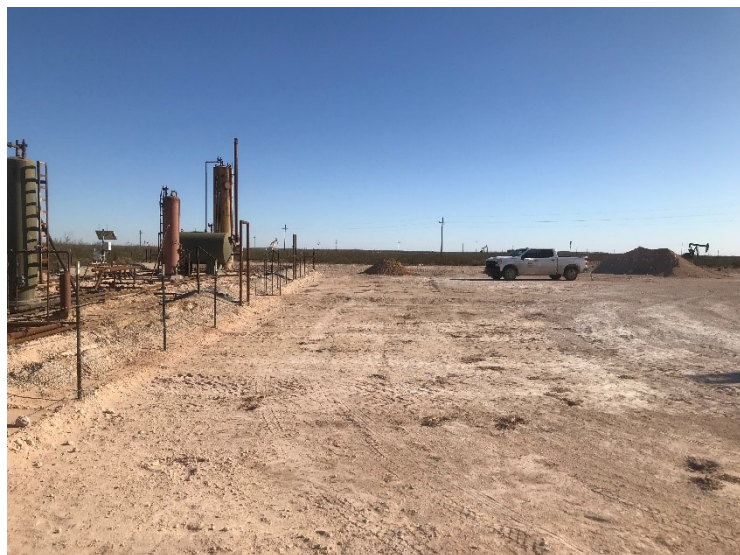
Photograph 11: Excavation south of containment.
