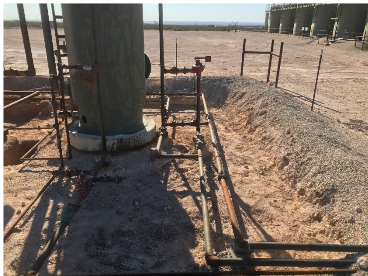
Photograph 9: Excavation around the heater treater release source.
