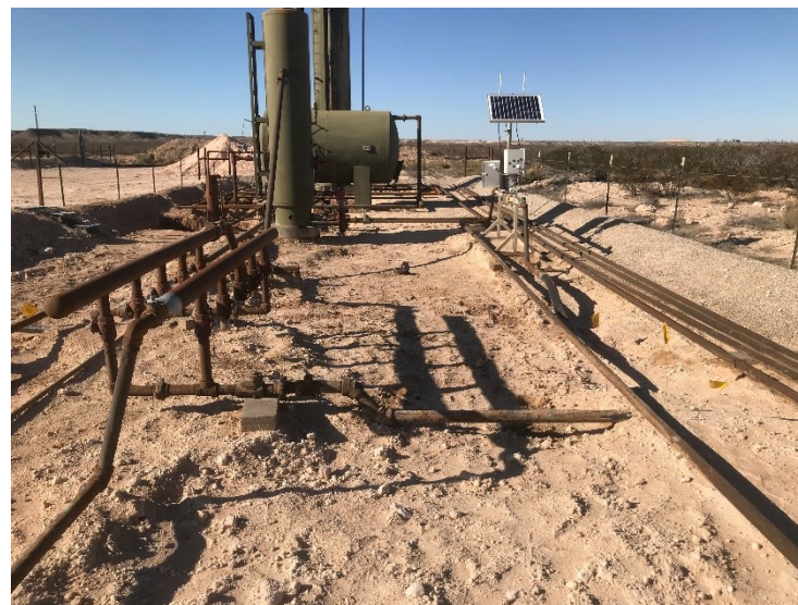
Photograph 6: Northwestern view within the containment.
