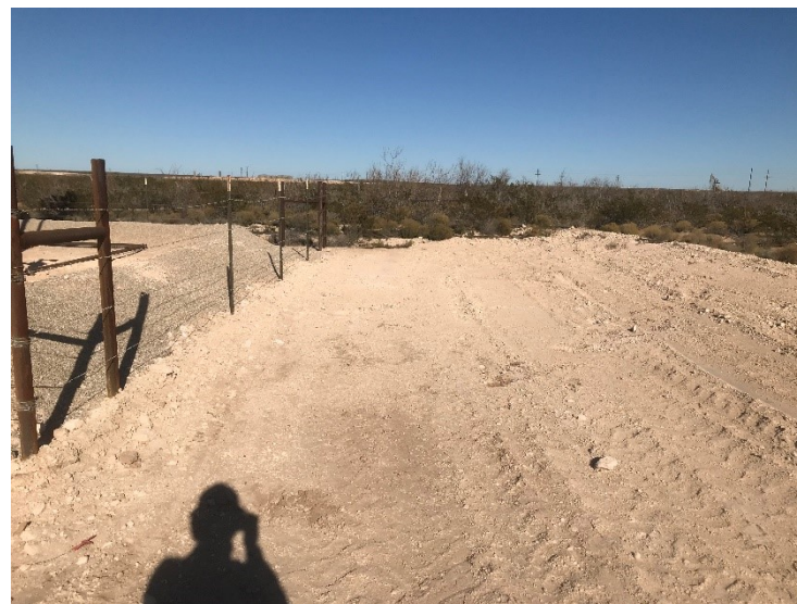
Photograph 10: Excavation southeast of containment.
