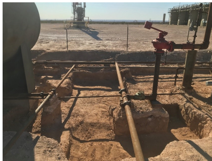
Photograph 8: Excavation within unlined secondary containment..
