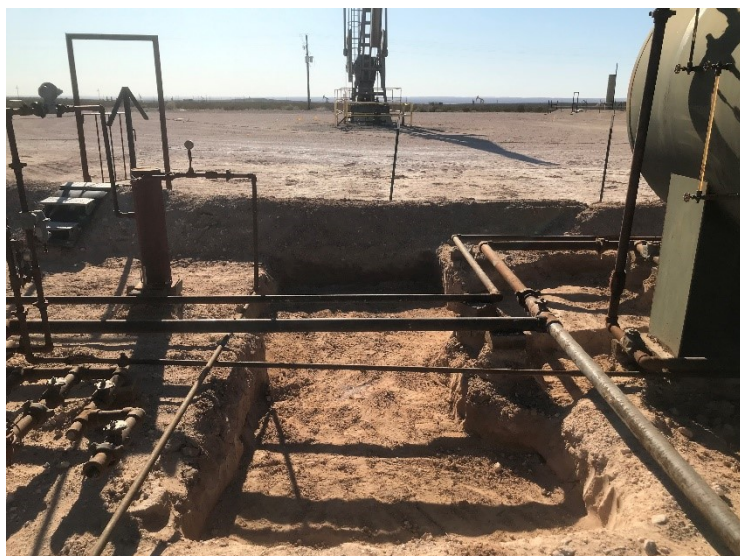
Photograph 7: Excavation within unlined secondary containment.
