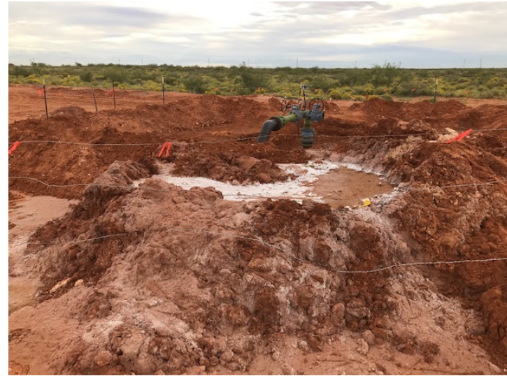
Photograph 2: East facing view of excavation surrounding release point.
