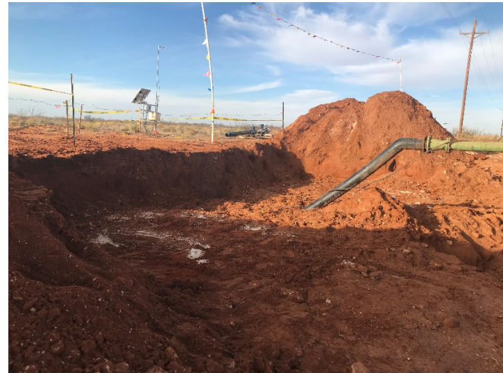
Photograph 4: Northwest facing view of final excavation.
