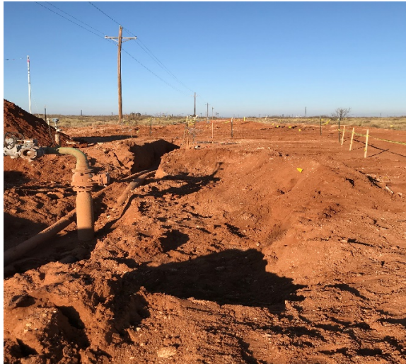
Photograph 3: North facing view of excavation surrounding release point.
