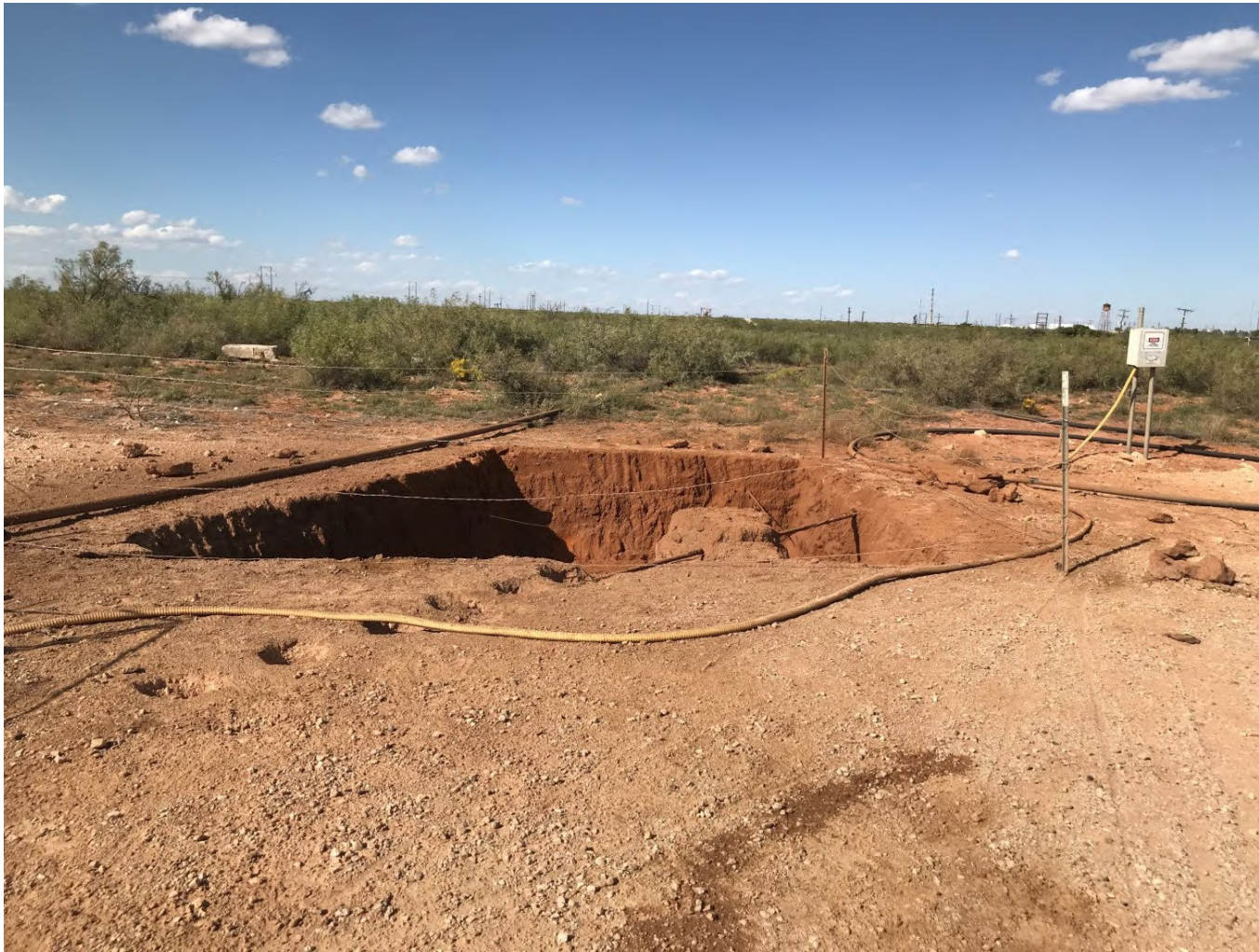
View of final western excavation extent during confirmation soil sampling activities facing north.
