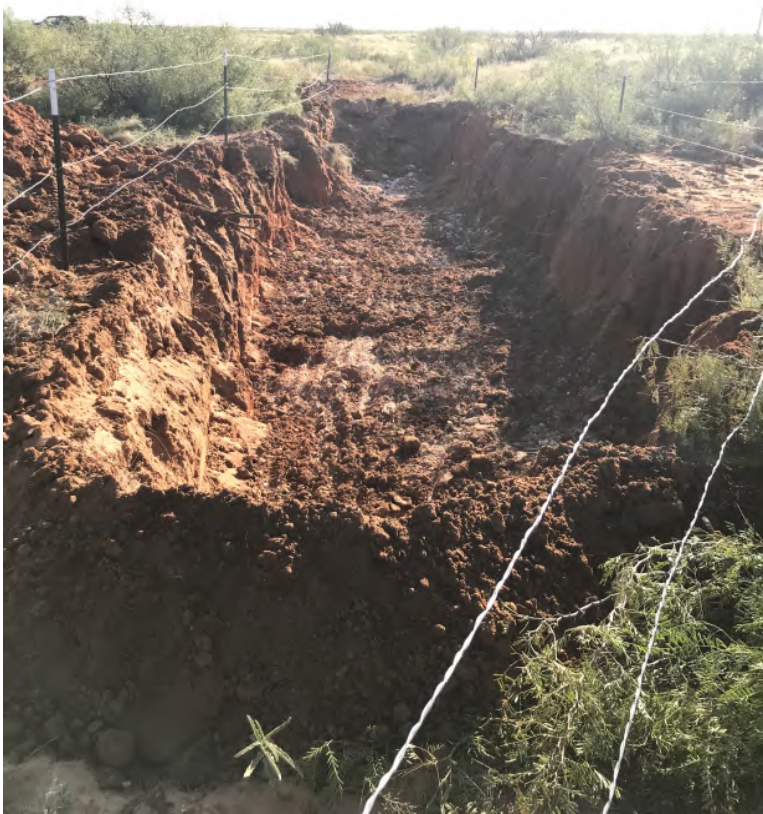
View of final southern excavation extent during confirmation soil sampling activities.
