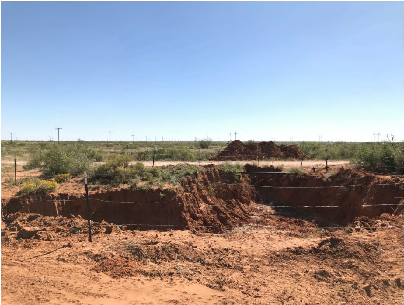
View of final northeastern excavation extent during confirmation soil sampling activities facing south.
