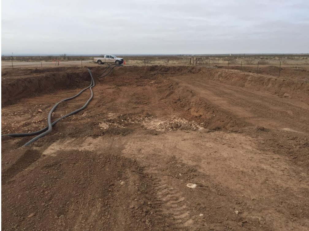
PHOTO 14: View of excavation, facing west. 11/08/2019
