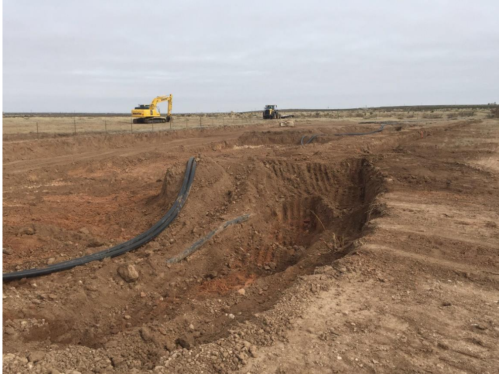
PHOTO 18: View of excavation, facing northeast. 11/08/2019
