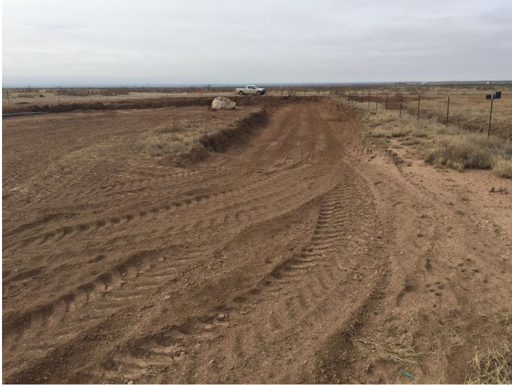
PHOTO 13: View of excavation, facing west. 11/08/2019
