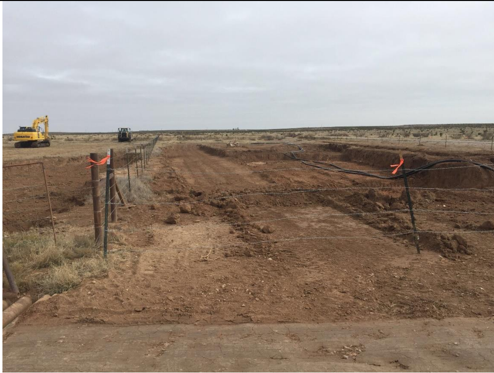
PHOTO 11: View of excavation, facing east. 11/08/2019
