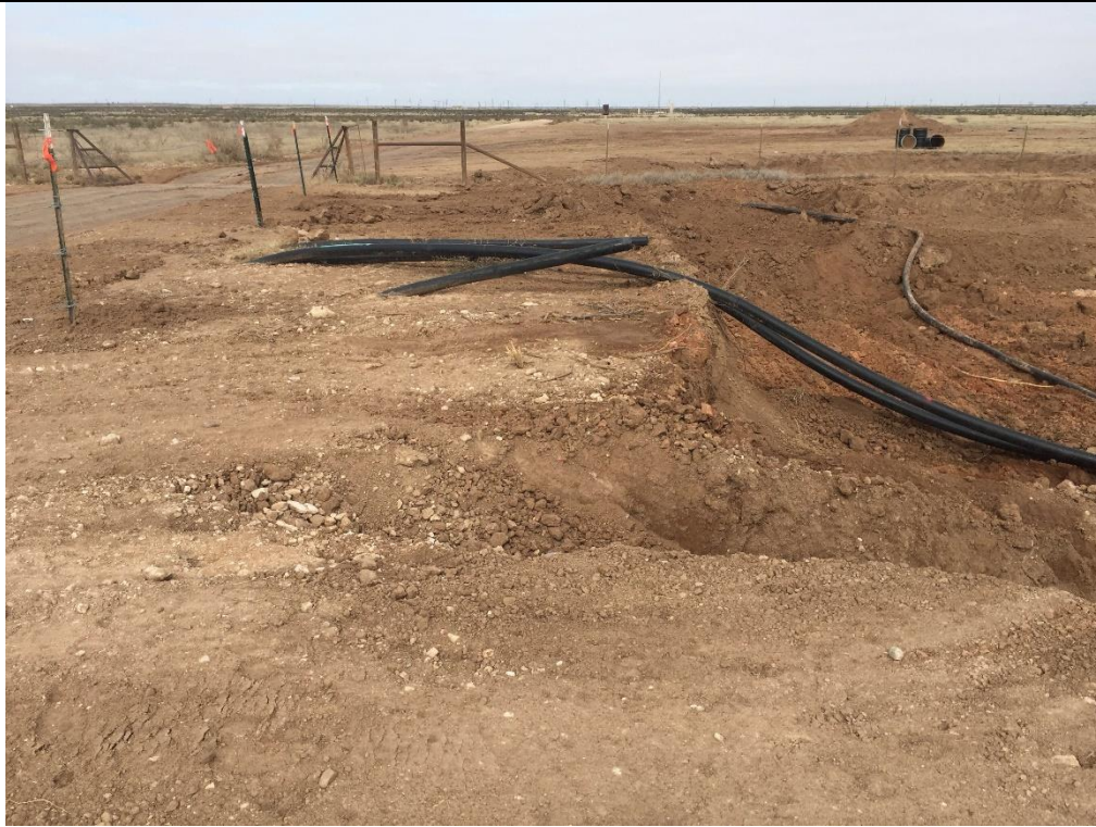
PHOTO 17: View of western portion of excavation, facing north. 11/08/2019
