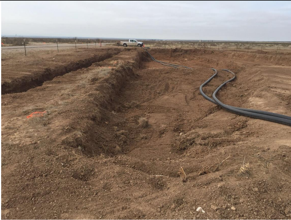
PHOTO 15: View of excavation, facing west. 11/08/2019
