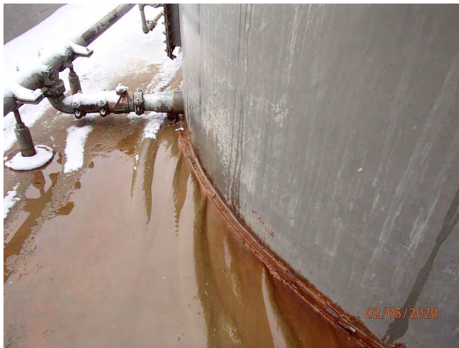
View of standing water and snow within the secondary containment.
