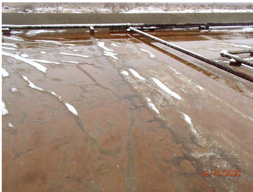
View of standing water in the secondary containment.
