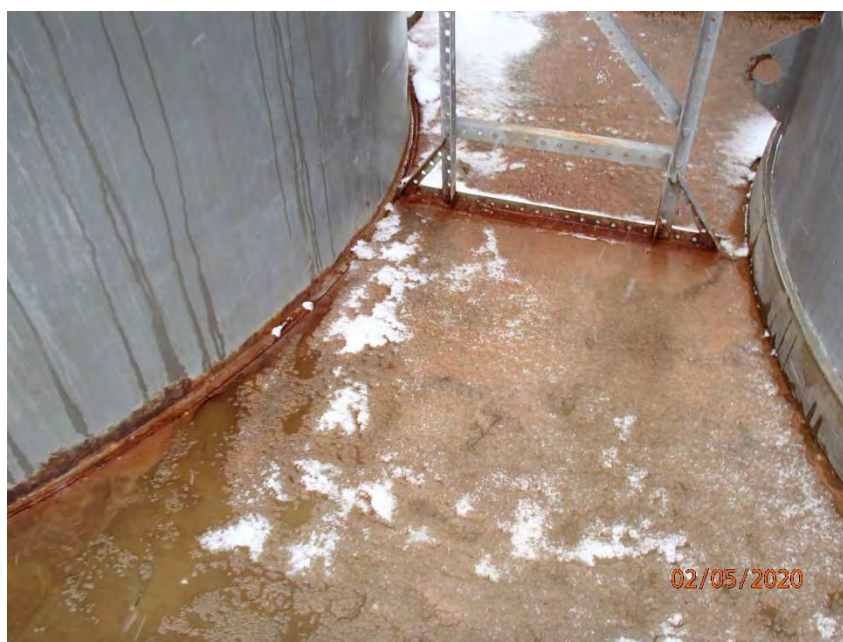
View of standing water between the tanks and rust on the bottom of the tank.
