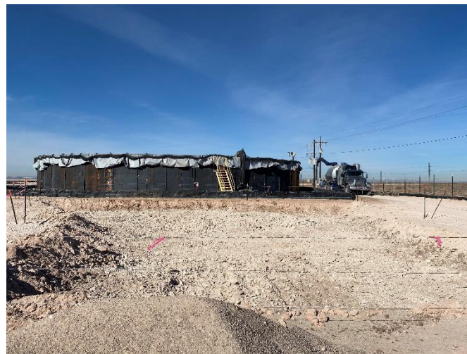
Photograph 3: View of excavation on east side of lined containment.
