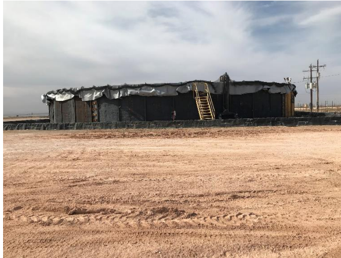
Photograph 2: View of east side of lined containment where overflow occurred.
