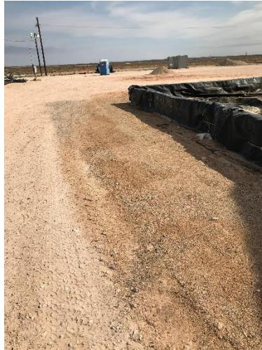
Photograph 1: View from north side of containment, facing east.
