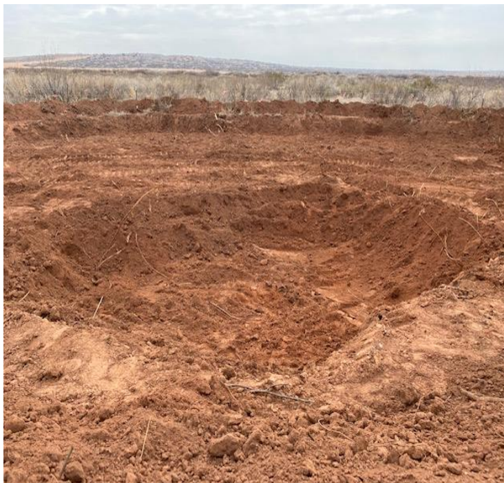
Photograph 5 Southern view of excavation during delineation activities.
