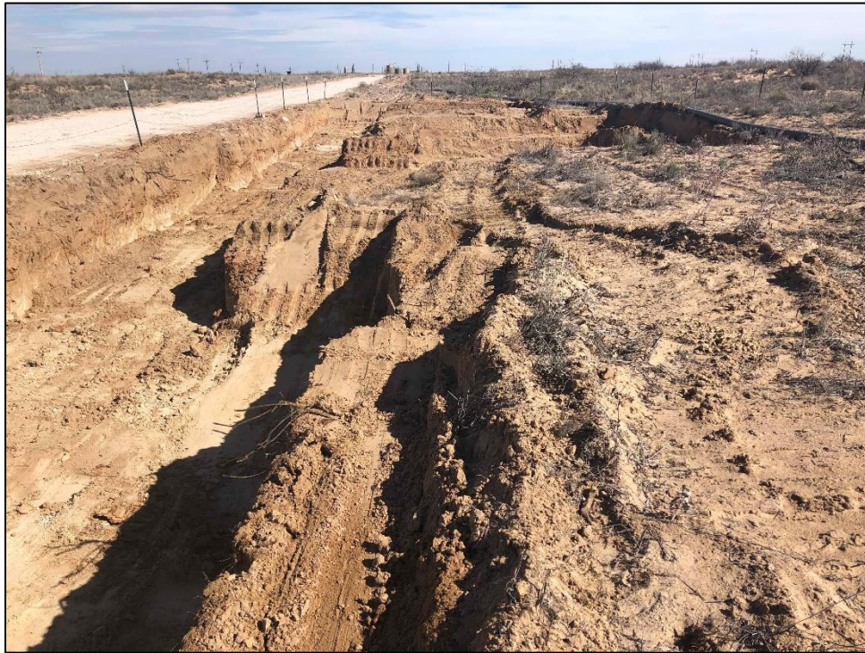
PHOTO 15: View of south of lease road excavation, facing east. 02/03/20 / TIME: 4:05PM / GPS: 32.6085 -103.4925
