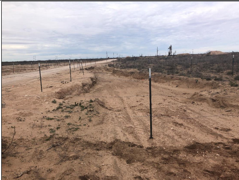
PHOTO 18: View of excavation north of lease road, facing west. 02/03/2019 / TIME: 11:51PM / GPS: 32.6085 -103.4925
