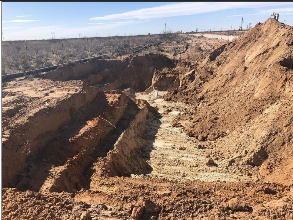
PHOTO 16: View of south of lease road excavation, facing west. 02/03/2020 / TIME: 4:00PM / GPS: 32.6085 -103.4925
