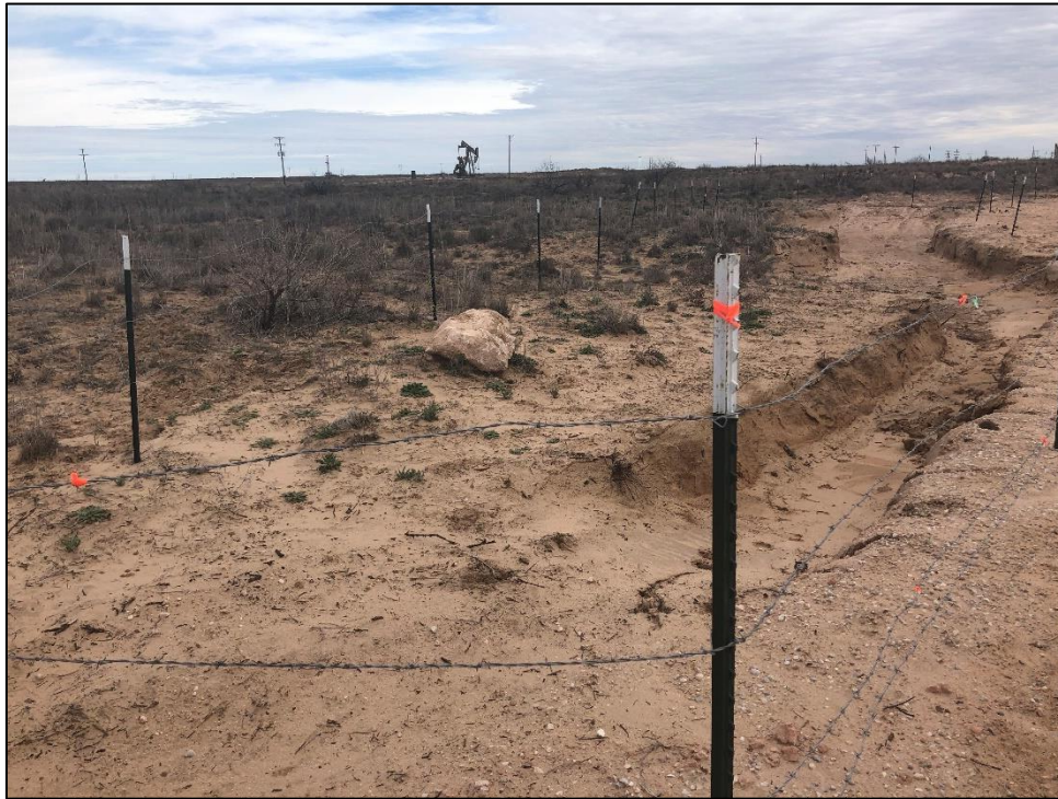
PHOTO 19: View of excavation north of lease road, facing east. 02/03/2019 / TIME: 11:52PM / GPS: 32.6085 -103.4925
