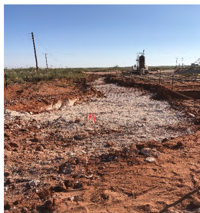
Photo #6 South facing view of excavation.
