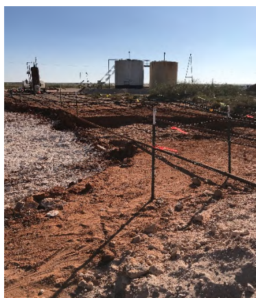
Photo #5 Southwest facing view of excavation.
