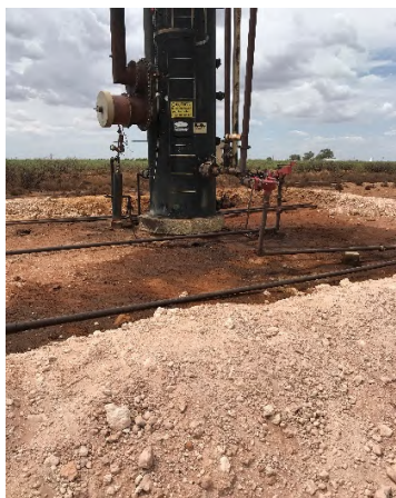
Photo #1 West facing view of spill within earthen berm.
