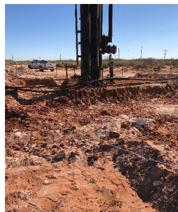
Photo #4 Southwest facing view of excavation near separator.
