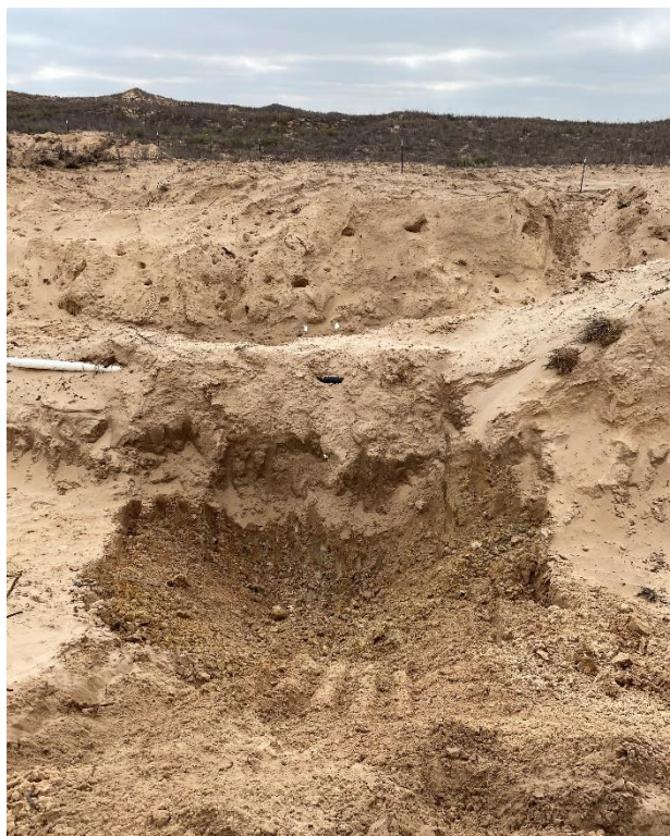
Southern view of final excavation extent in during confirmation soil sampling activities.
