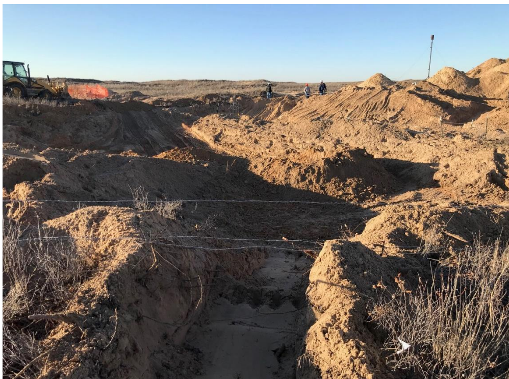
Northwestern view of final excavation extent during confirmation soil sampling activities.
