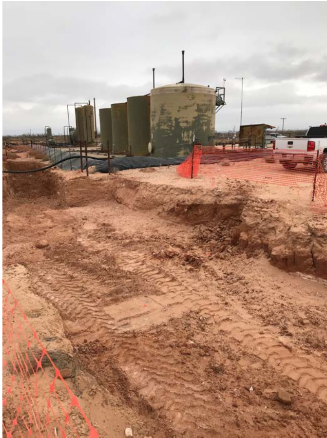
View of Excavation
