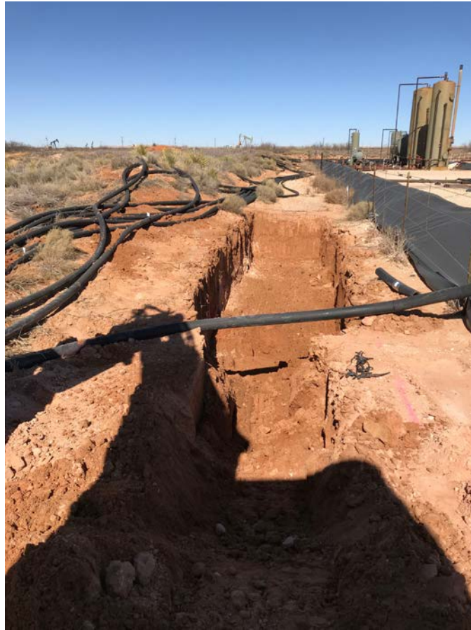
View North of Excavation
