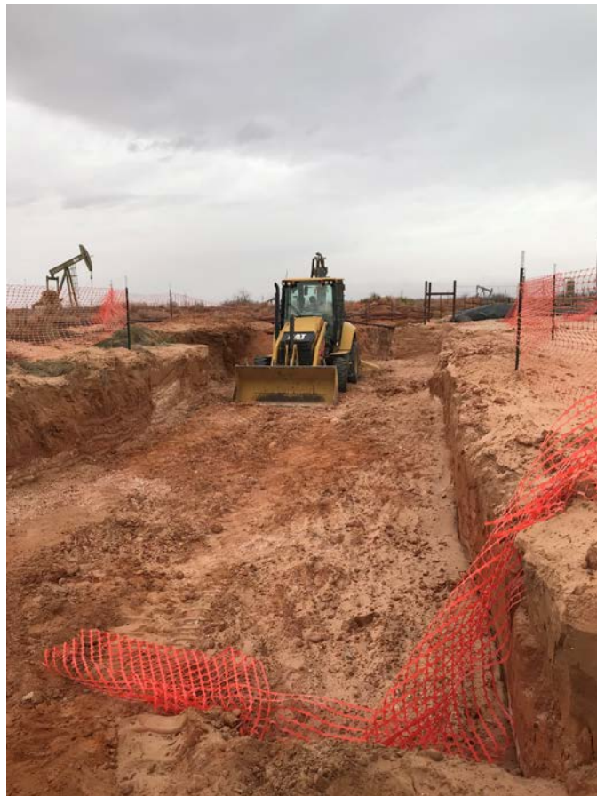
View South of Excavation
