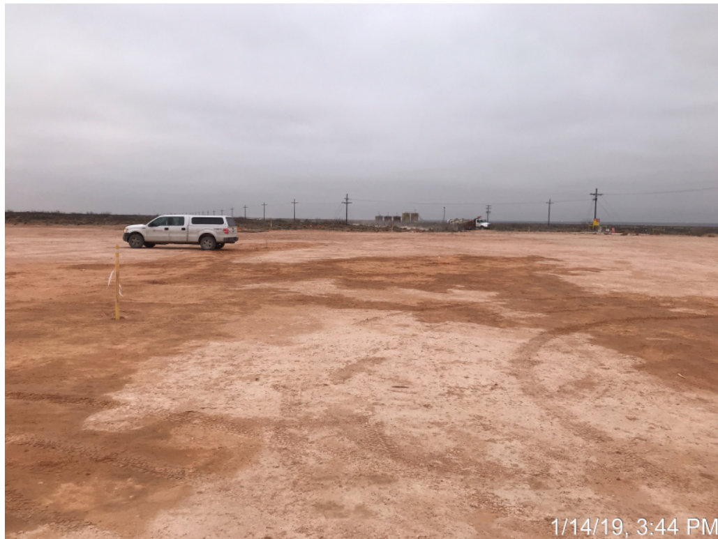
Area of AH-5 – View to North
