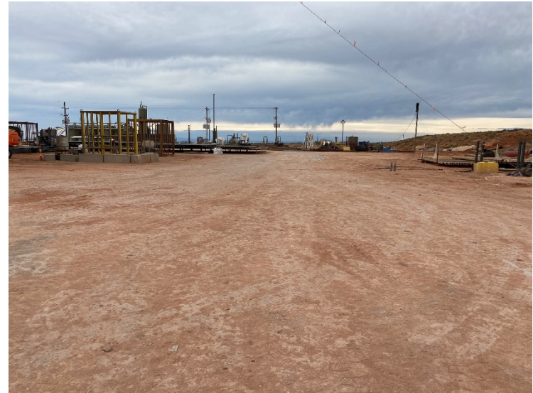
Photograph 4: View of equipment on Site facing west.
