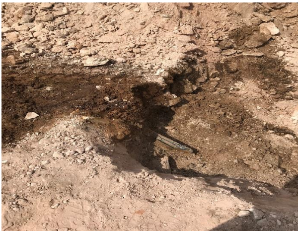
Line Strike in Test Trench
