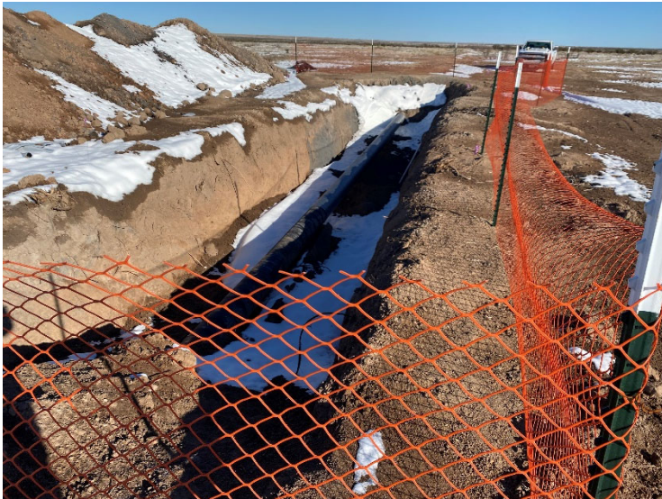
Photograph 3: View of the Site facing north.
