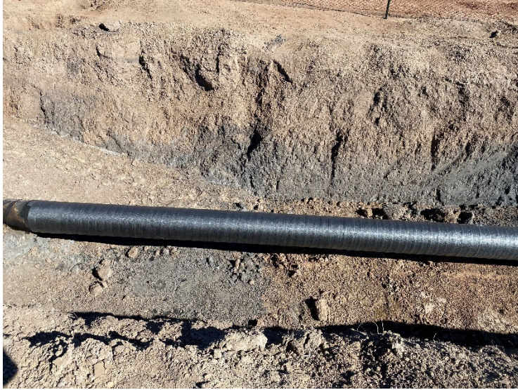
Photograph 5: View of the repaired subsurface flowline.
