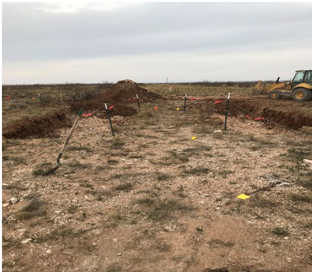
Photograph 3: Northern view of excavation extent.
