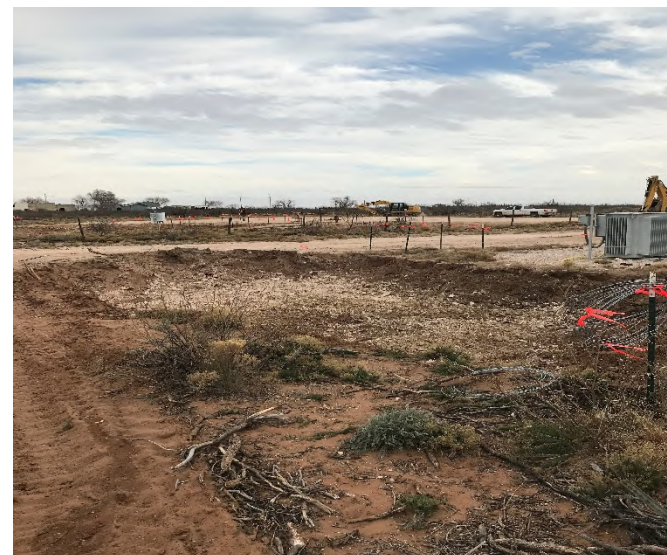
Photograph 4: Eastern view of excavation extent.
