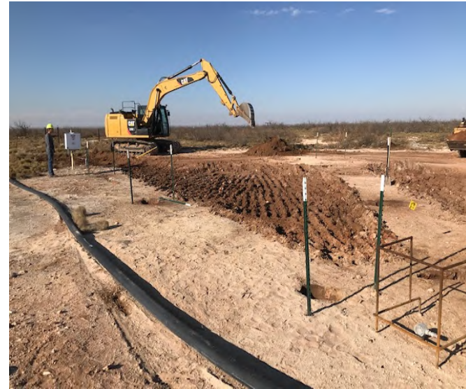
Photograph 2: Northwest view of on pad excavation extent.
