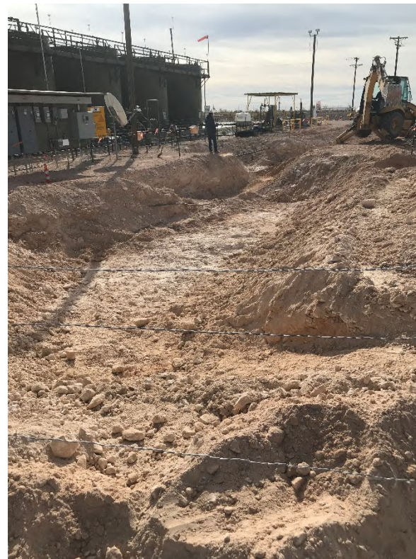
Photograph 4: South facing view of excavation.
