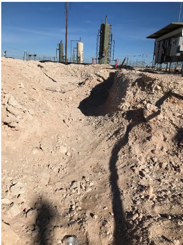
Photograph 3: North facing view of excavation.
