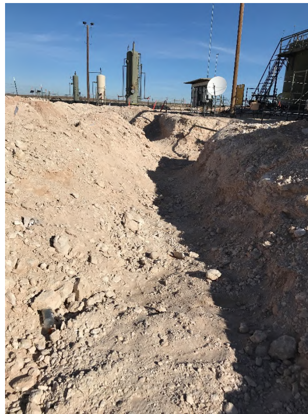
Photograph 2: North facing view of excavation.
