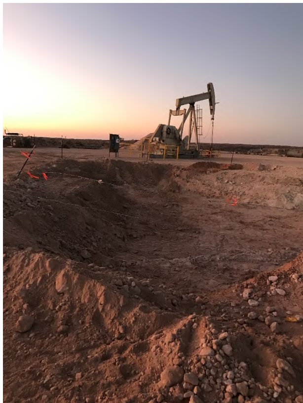
Photograph 1: Northwest facing view of excavation.
