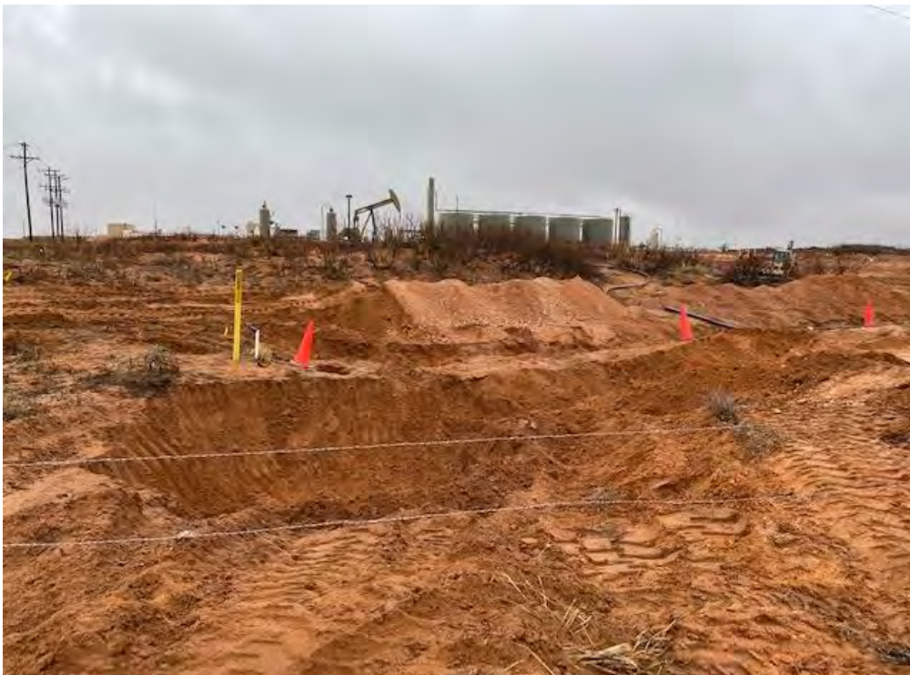
Northern view of excavation in the pasture area during confirmation soil sampling activities.
