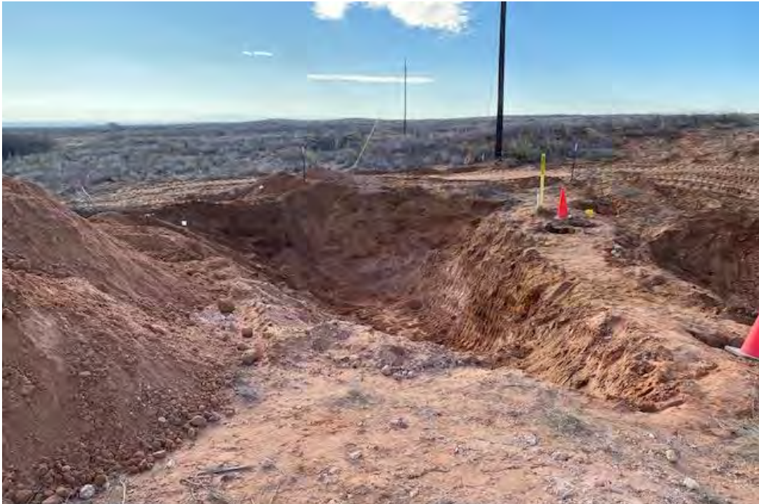
Western view of southern excavation extent during confirmation soil sampling activities.
