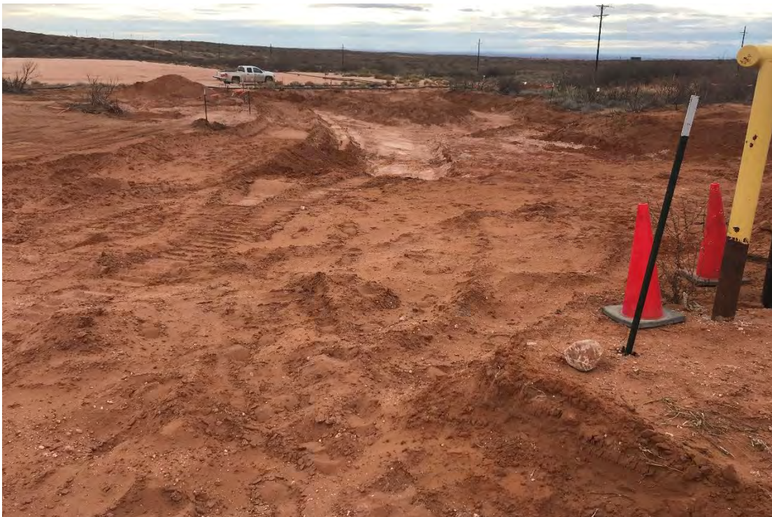
Southern view of excavation in the pasture area during excavation activities.
