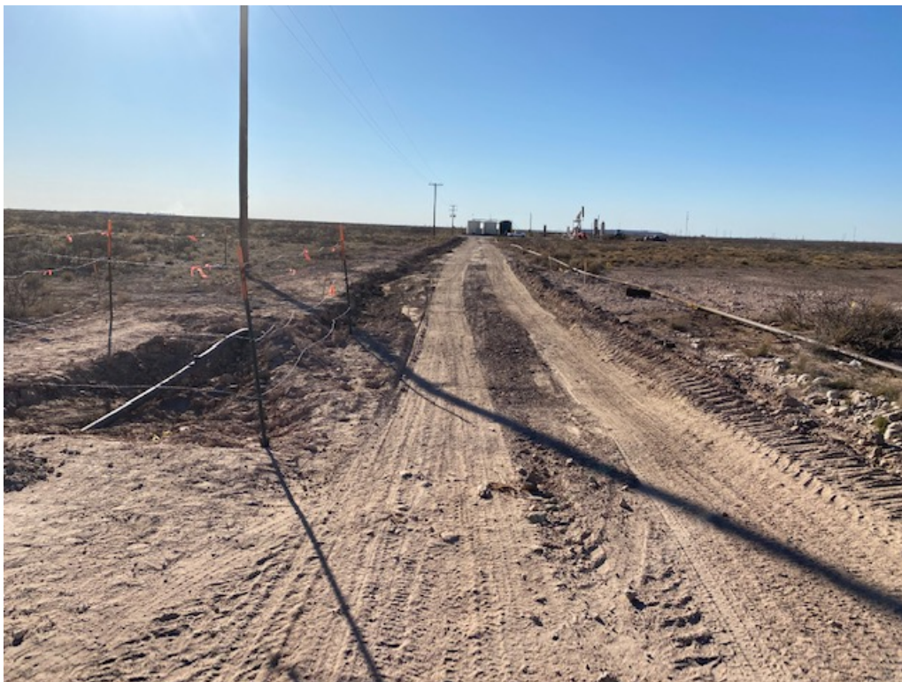
Photograph 3: View of excavation along lease road facing west.
