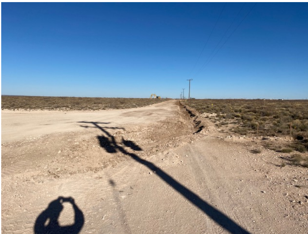
Photograph 4: View of excavation along lease road facing east.
