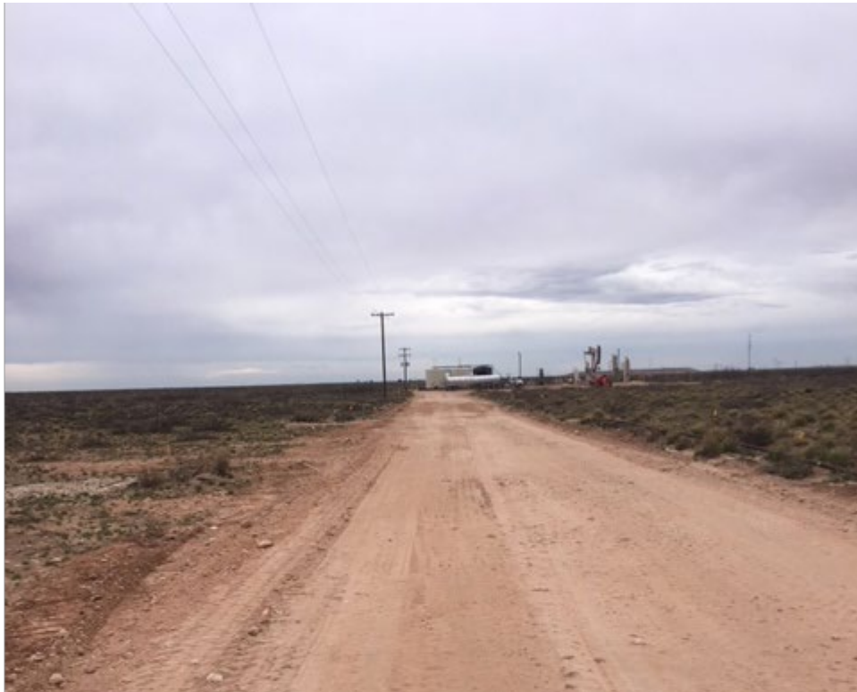
Photograph 6: View of post-compacted backfill on lease road facing west.
