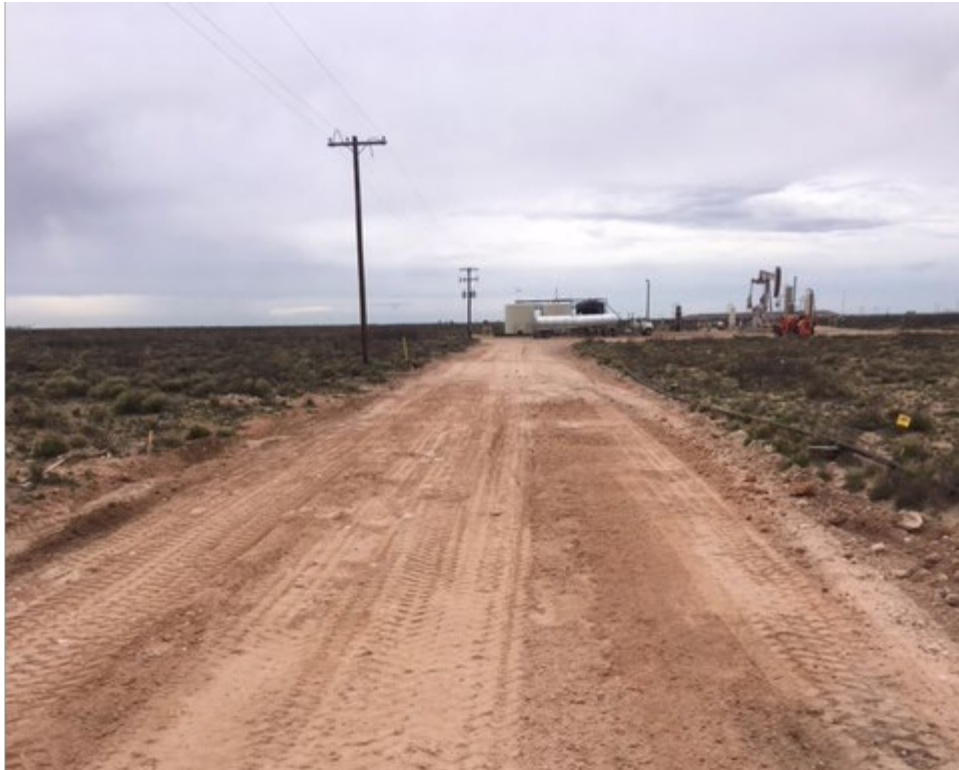
Photograph 5: View of pre-compacted backfill on lease road facing west.
