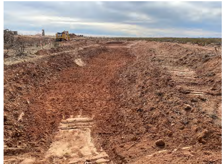
Photograph 4: View of excavation extent facing west.
