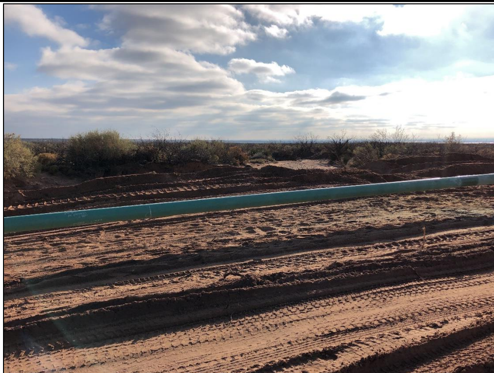
PHOTO 27: View of HS-4, facing south. 12/25/2019 / TIME: 2:00PM / GPS: 32.0066, -103.8292
