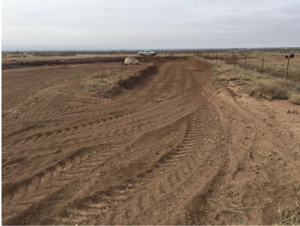
PHOTO 13: View of excavation, facing west. 11/08/2019
