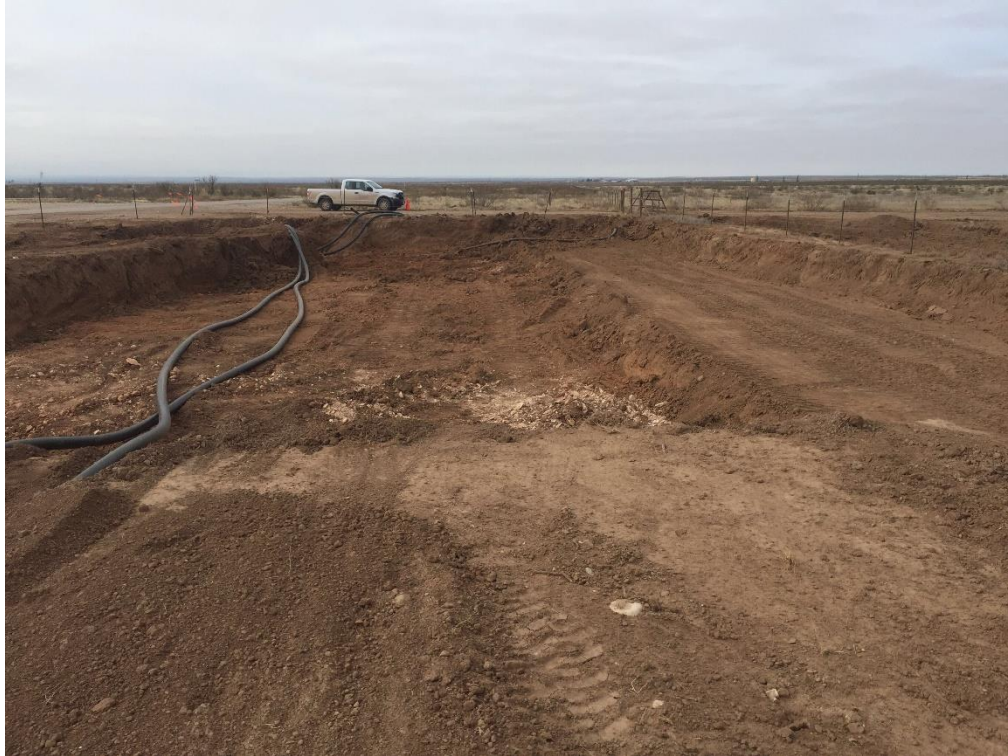
PHOTO 14: View of excavation, facing west. 11/08/2019
