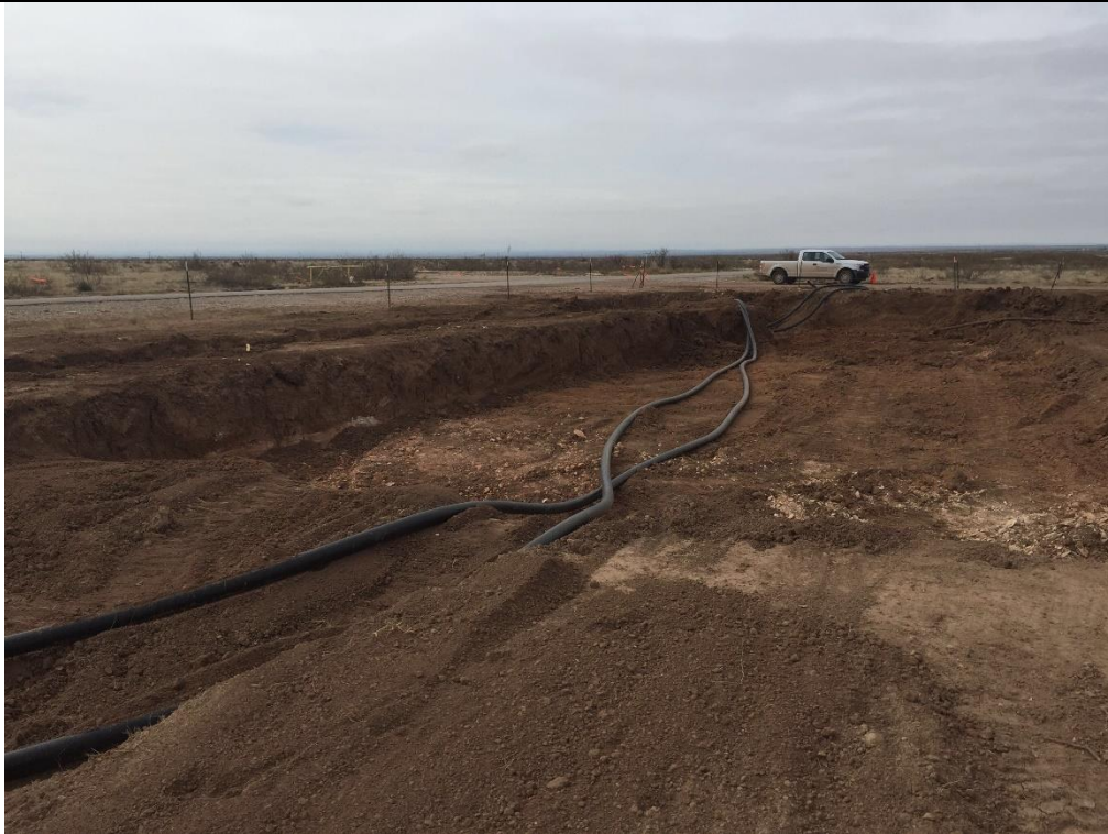
PHOTO 16: View of excavation, facing southwest. 11/08/2019
