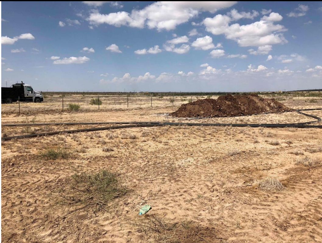
PHOTO 3: View of stockpile, facing North. 8/14/2019
