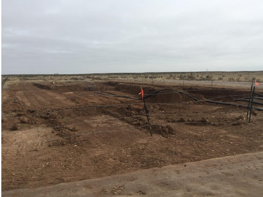
PHOTO 12: View of excavation, facing southeast. 11/08/2019
