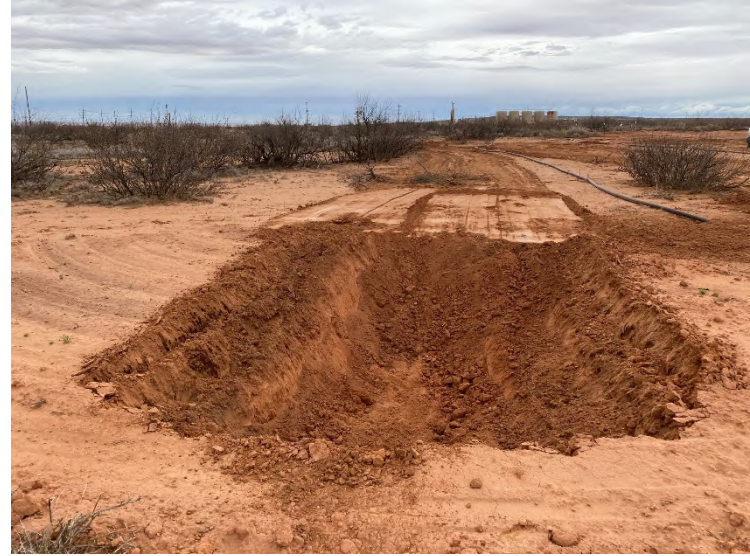
Photograph 2: Northern view of excavated PH07 area.
