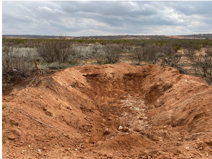
Photograph 3: Southern view of excavated PH10 area.
