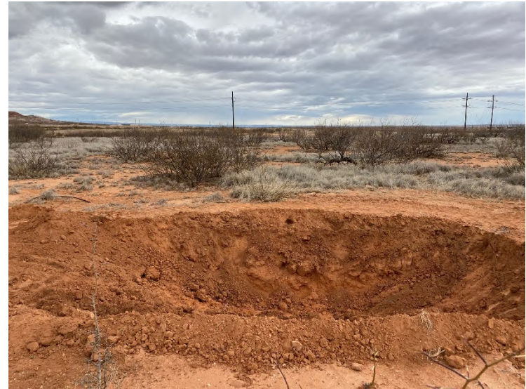
Photograph 4: Western view of excavated PH06 area.
