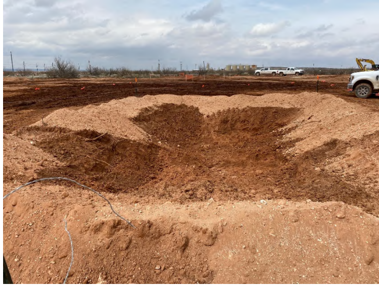
Photograph 1: Northern view of excavated PH04 area.
