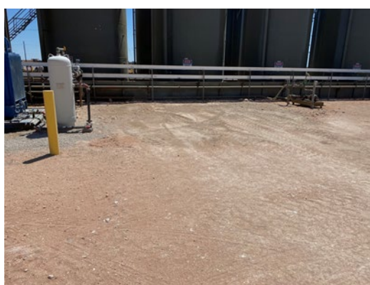
Photograph 6: View of final backfill.
