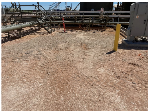
Photograph 5: View of final backfill.
