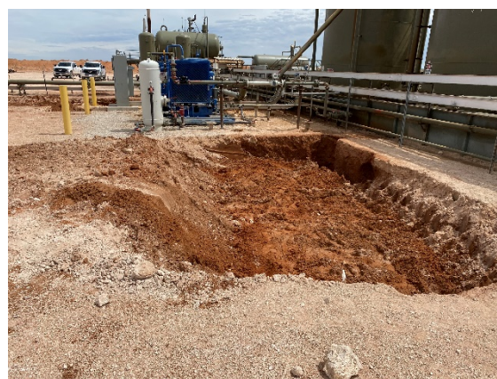
Photograph 4: View of excavation facing east.
