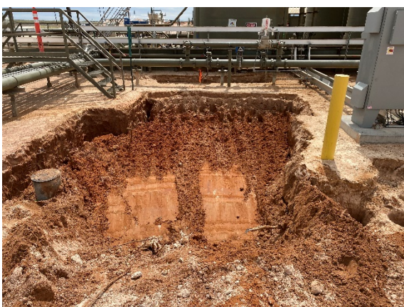
Photograph 3: View of excavation between active equipment facing south.
