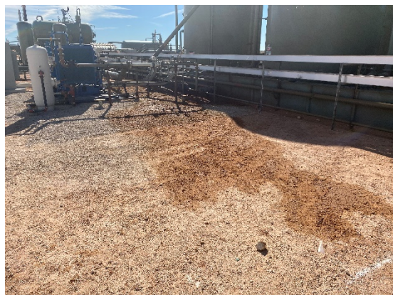
Photograph 2: View of staining north of lined containment on pad.
