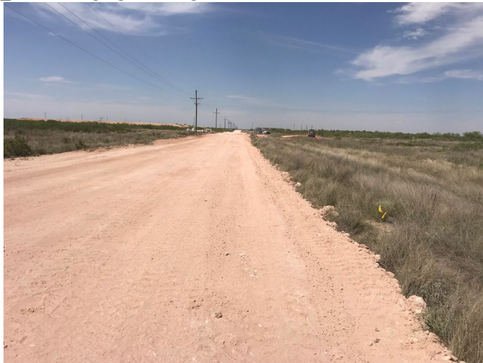
COG_PG14: Backfill - View from south
