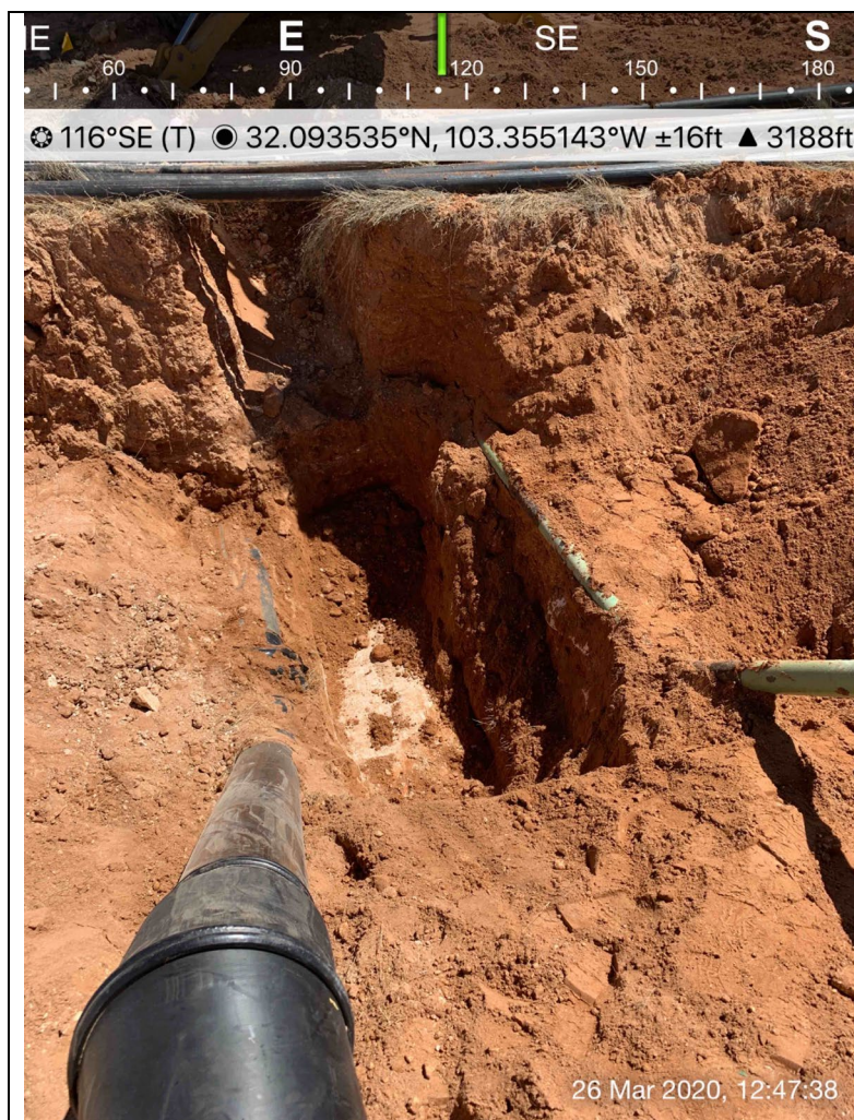
COG_PG03: View of initial remediation excavation near pipelines
