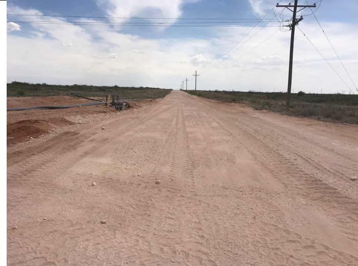
COG_PG14: Backfill - View from north
