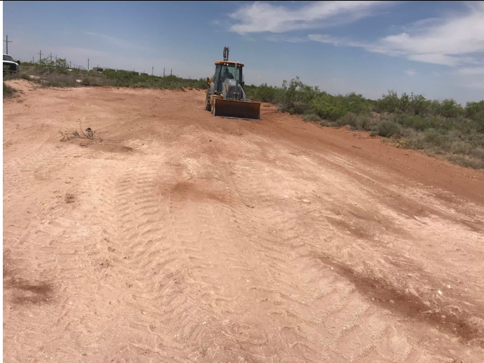
COG_PG13: Staging/Loading area - Post backfill
