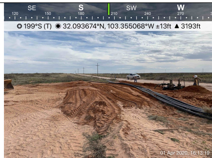
COG_PG10: Initial excavation backfill activities.
