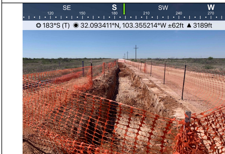
COG_PG11: View of road excavation (North to South)
