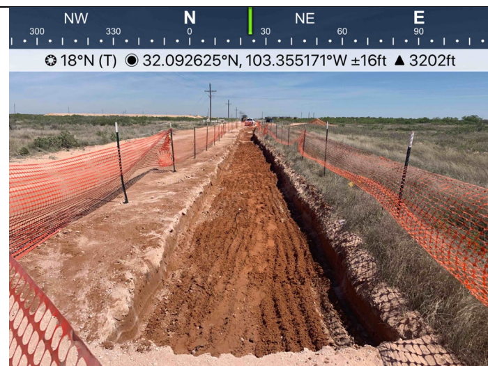
COG_PG12: View of road excavation (South to North)
