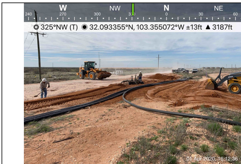
COG_PG09: Initial excavation backfill activities
