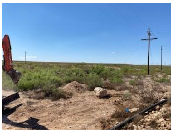
Photograph 18: Potholing north of the release extent.
