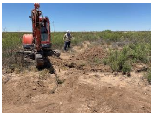
Photograph 16: Northwestern view of potholing north of the release extent.
