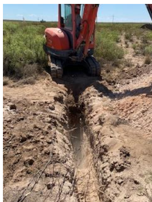
Photograph 17: Potholing north of the release extent (PH18).
