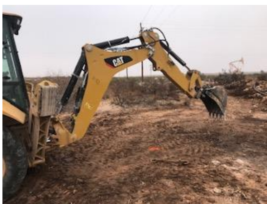
Photograph 17: Potholing within the pasture release extent.
