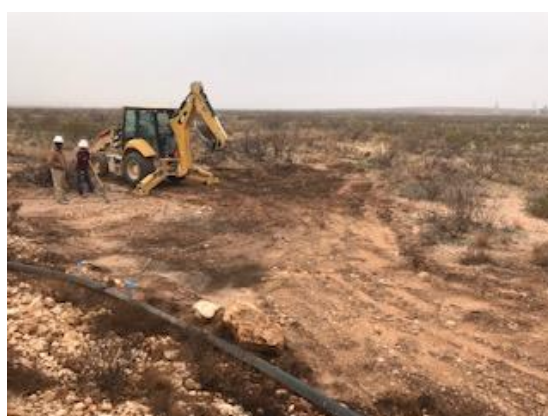
Photograph 18: Potholing within the pasture release extent.
