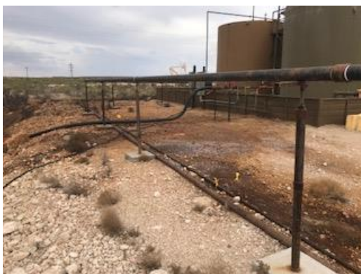
Photograph 1: Northeastern view of the release extent on pad.
